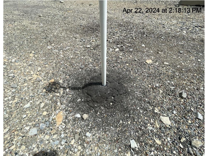
Photo # 4675 Stained soils & gravel
