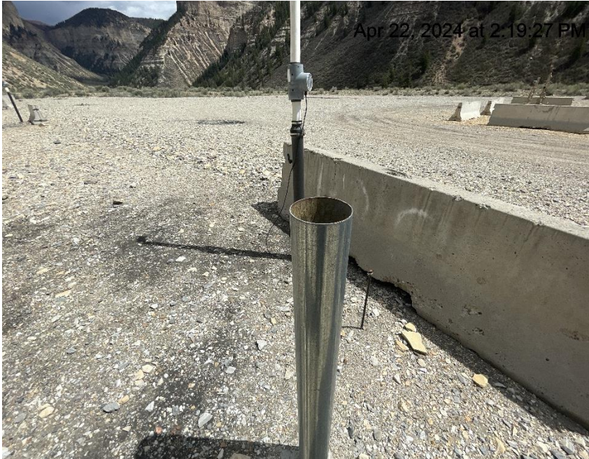
Photo # 4656 Open ended piping/wildlife hazard
