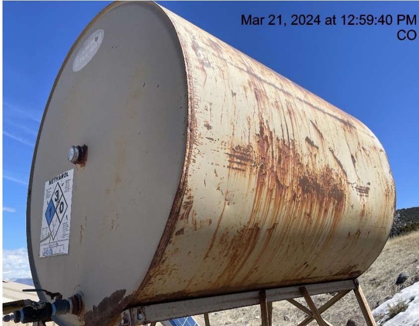
Photo # 988 From inspection 708903378 conducted on 03/21/2024 Methanol tank improperly labeled/lacks required information
