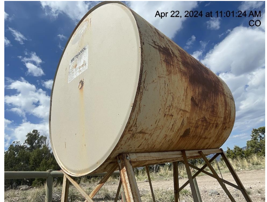
Photo # 4575 Methanol tank improperly labeled/lacks required information
