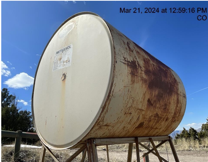
Photo # 987 From inspection 708903378 conducted on 03/21/2024 Methanol tank improperly labeled/lacks required information
