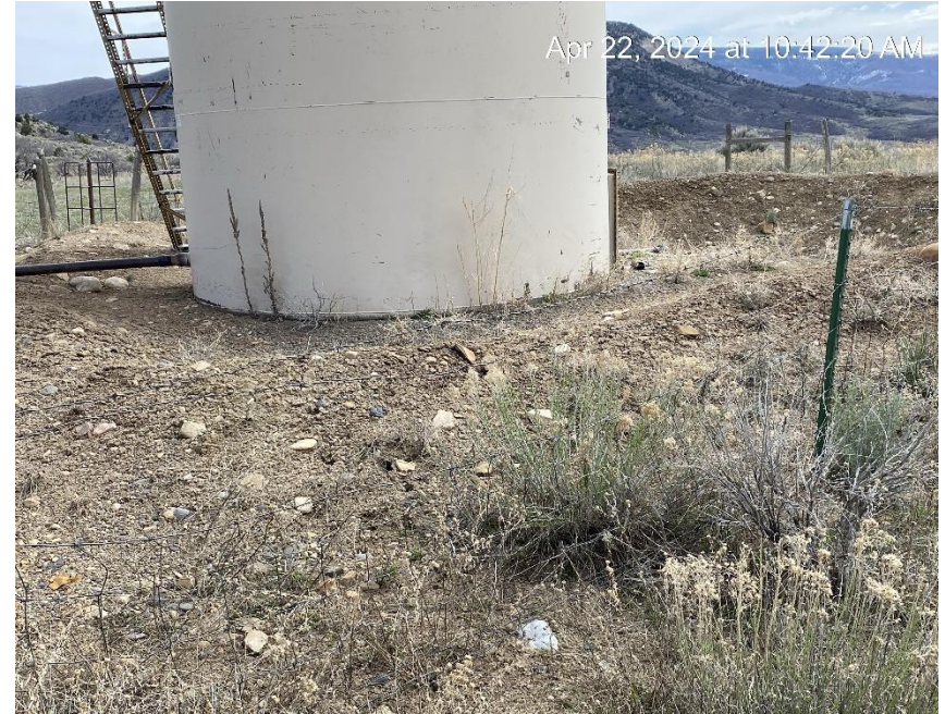
Berm not able to hold 150% of tank capacity
