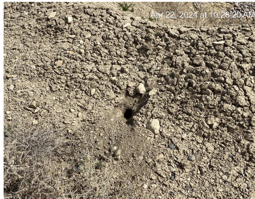
Burrow in earth tank berm.
