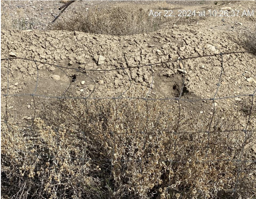
Burrowing in earth tank berm.
