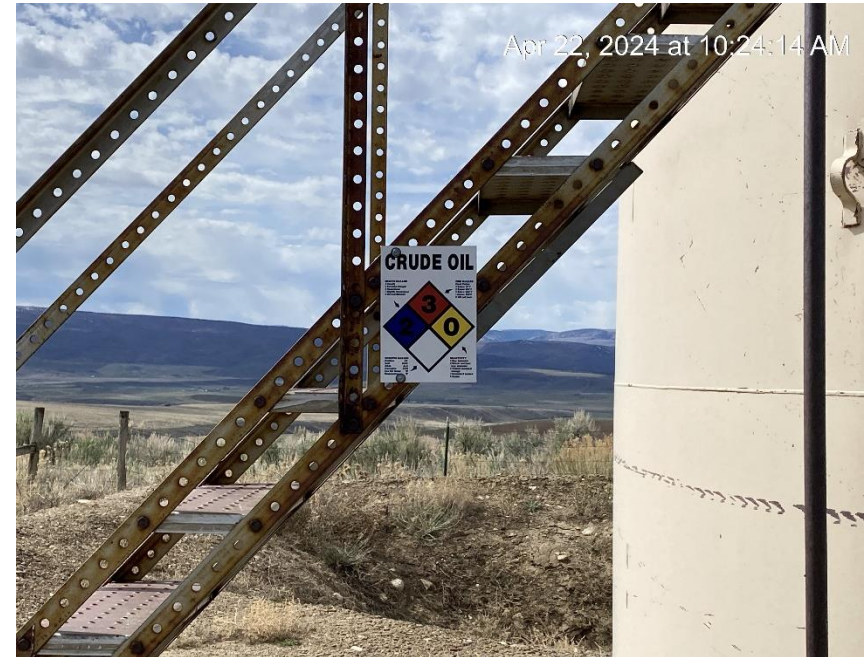
Tank labeling inadequate
