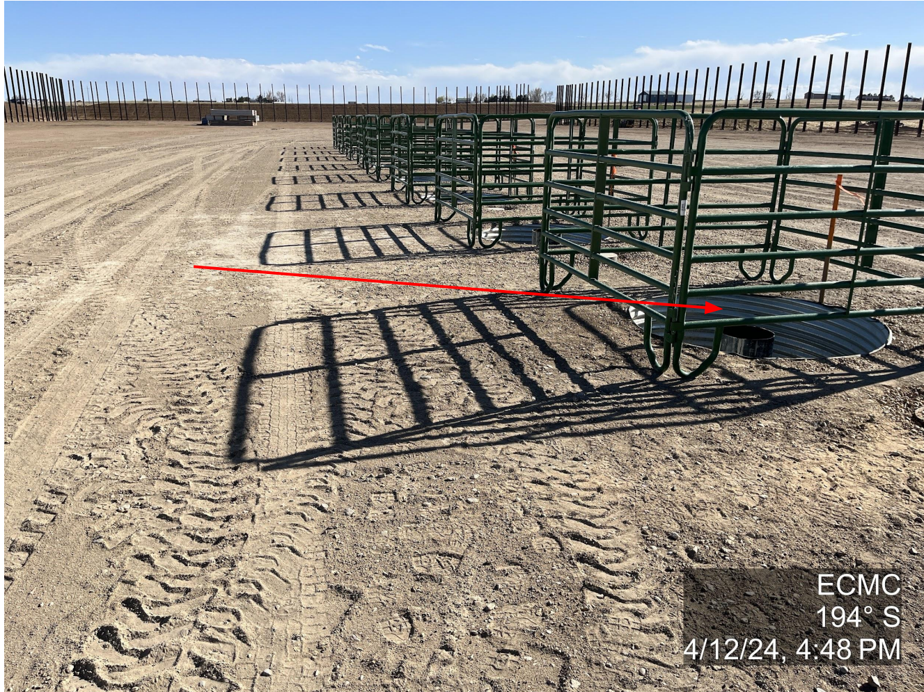
Photo 13. The photo was taken at the well location facing South. The photo illustrates that the operator has failed to install night caps on the surface casings.
