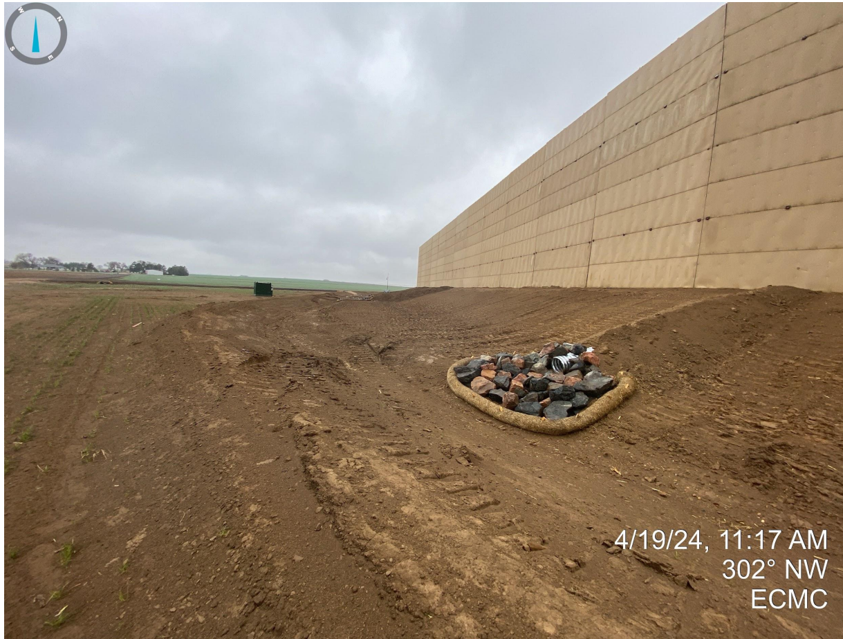
Photo 12. Taken near the southern/southeastern portion of the disturbance area. Photo illustrates outlet protections and unstabilized soils within the ditch and berm and slopes. Additional stabilization BMPs are required on the bare/exposed soils.
