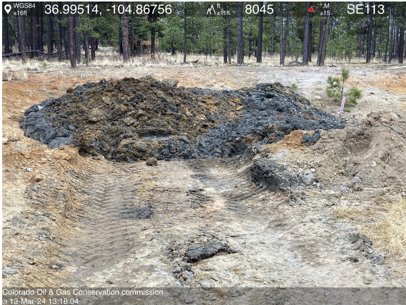
PHOTO 5: IT APPEARS THAT THE PRODUCED WATER PIT HAS BEEN CLEANED AND THE SECONDARY CONTAINMENT FOR THE PIT MATERIAL STORED ON LOCATION HAS BEEN COMPROMIZED AND THERE IS NO RUN ON PROTECTION IN PLACE TO PREVENT STORM WATER FROM MIXING WITH PIT MATERIAL. INTALL AND REPAIR BERMS PER 1002 SERIES RULES. CA DATE 5-22-2024.
