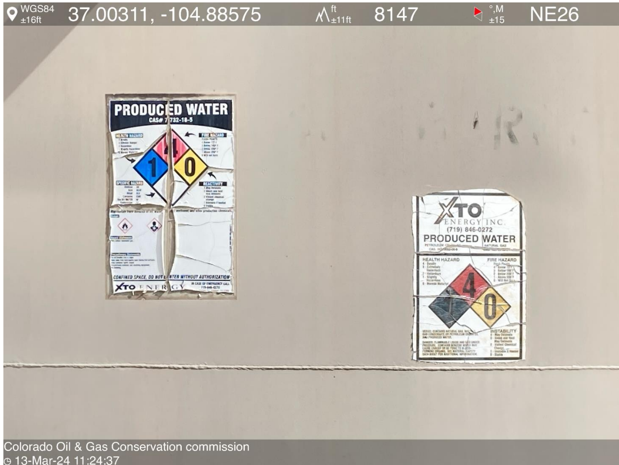
PHOTO 5: NOTE NFPA STICKERS ARE STILL LABELED WITH OLD OPERATOR WITH AN OLD PHONE NUMBER POSTED. Install sign to comply with Rule 605.h. (OLD OPERATOR EMERGENCY CONTACT NUMBERS SHALL NOT BE POST ON LOCATION.) CA DATE 5-22-2024.
