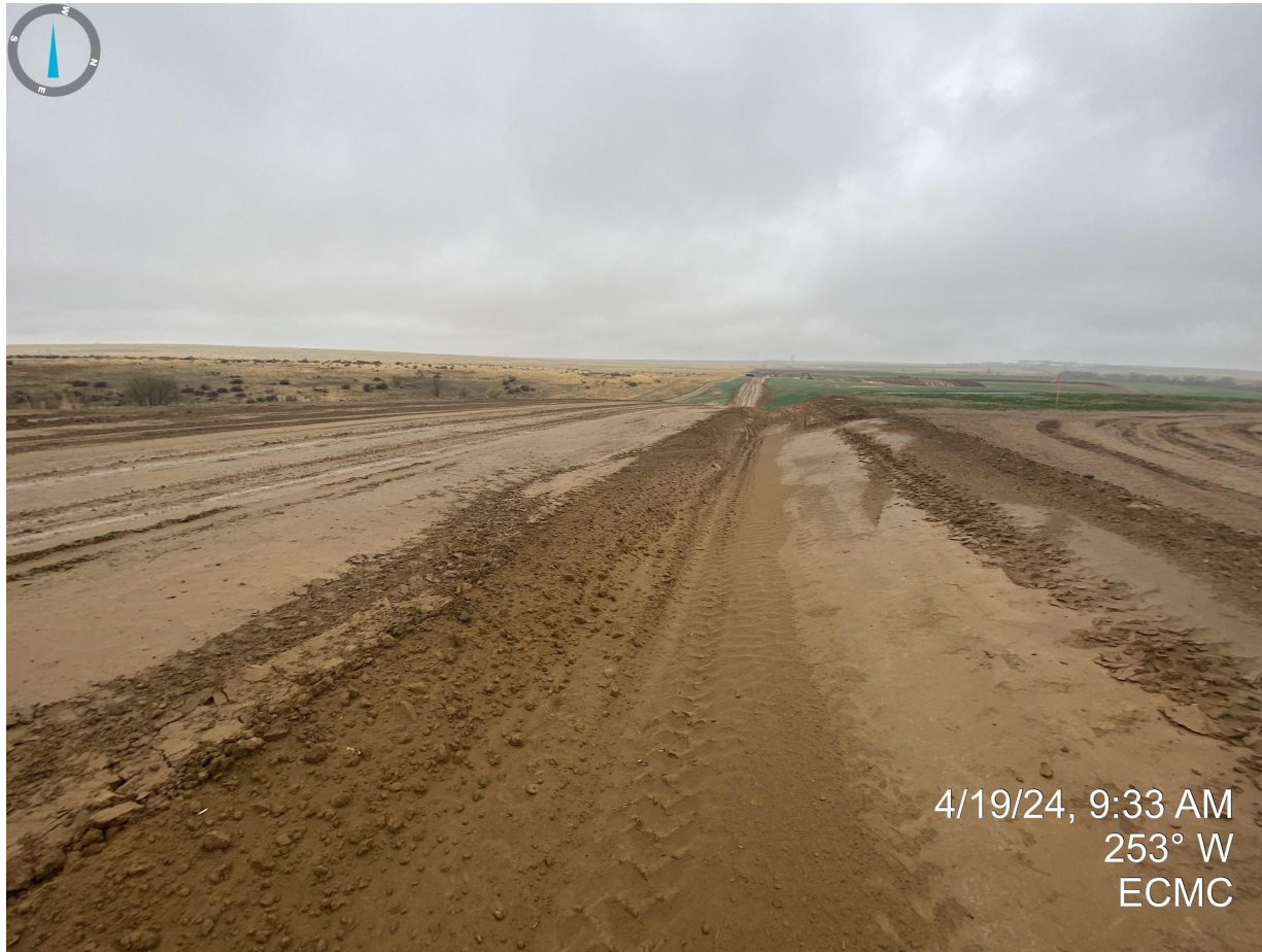
Photo 1. Taken near the start of the access road, facing west. It appears that topsoil has been salvaged and a stormwater ditch has been constructed.
