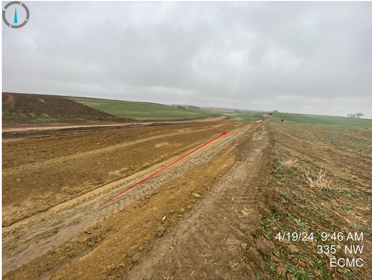
Photo 4. Stormwater ditch constructed along the east side of the disturbance area.
