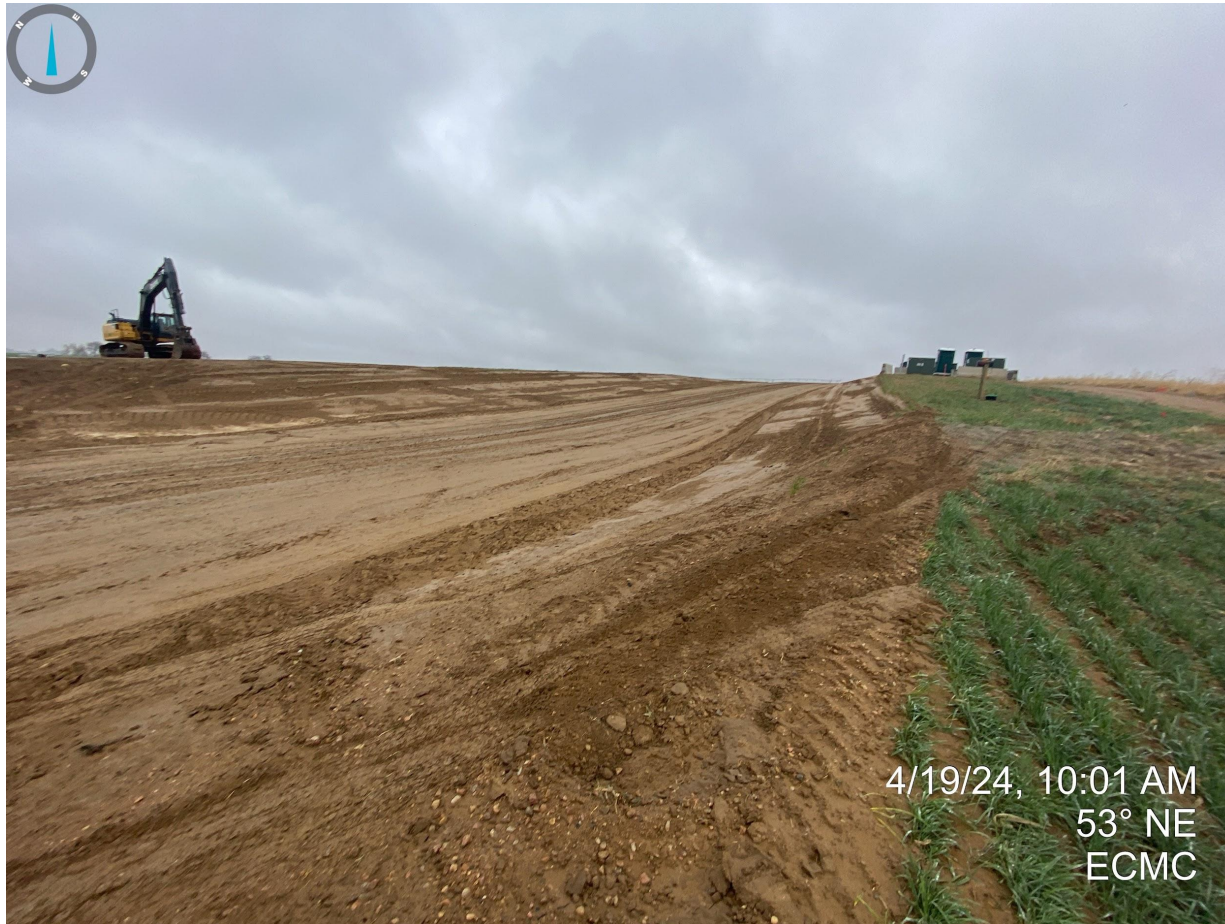
Photo 12. Looking northeast along the access road start from the disturbance area. It appears that topsoil has been salvaged and a stormwater ditch has been constructed.
