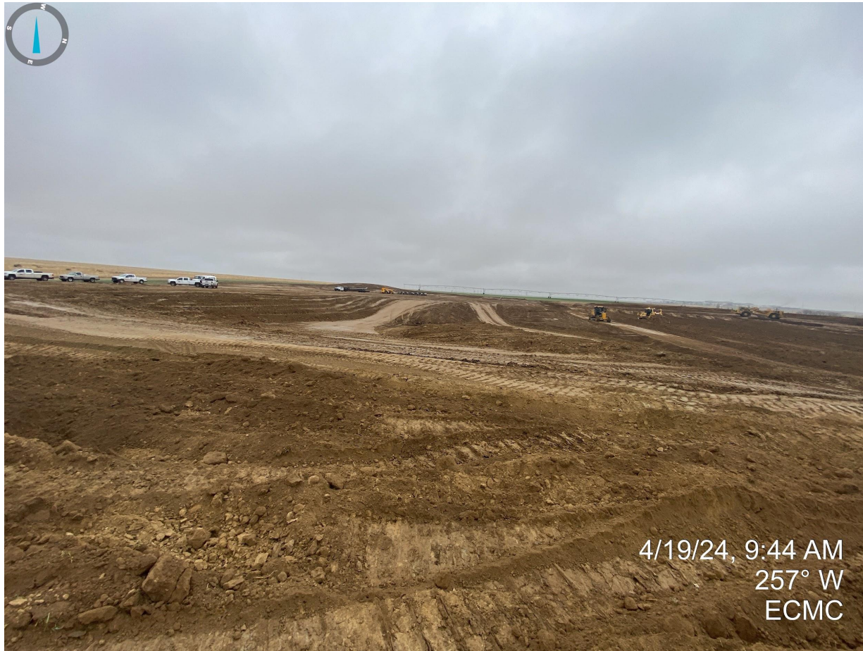
Photo 2. Taken near the east side of the disturbance area. Photo illustrates topsoil salvage activities and cut/fill operations.
