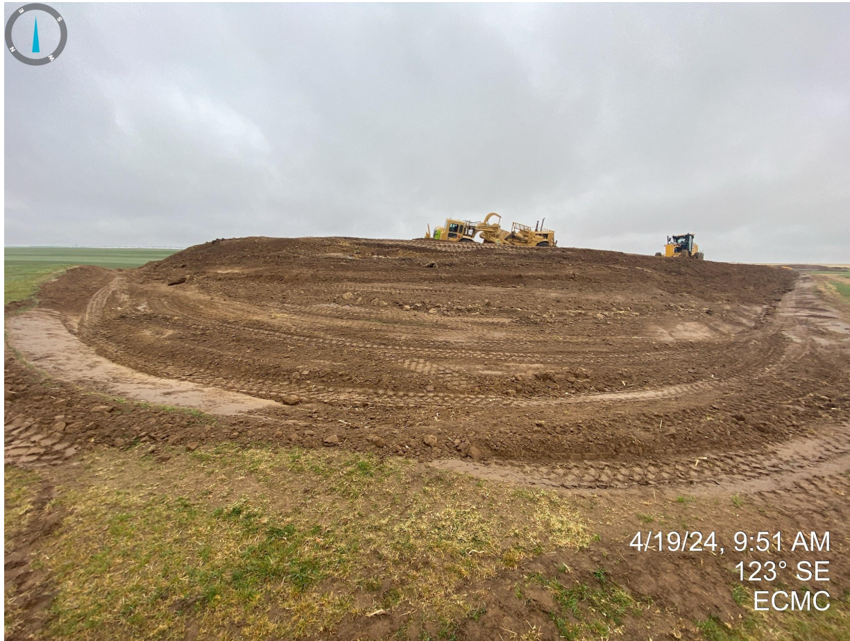
Photo 7. Taken near the northwest corner of the disturbance area. Topsoil salvage activities were ongoing at the time of this inspection.
