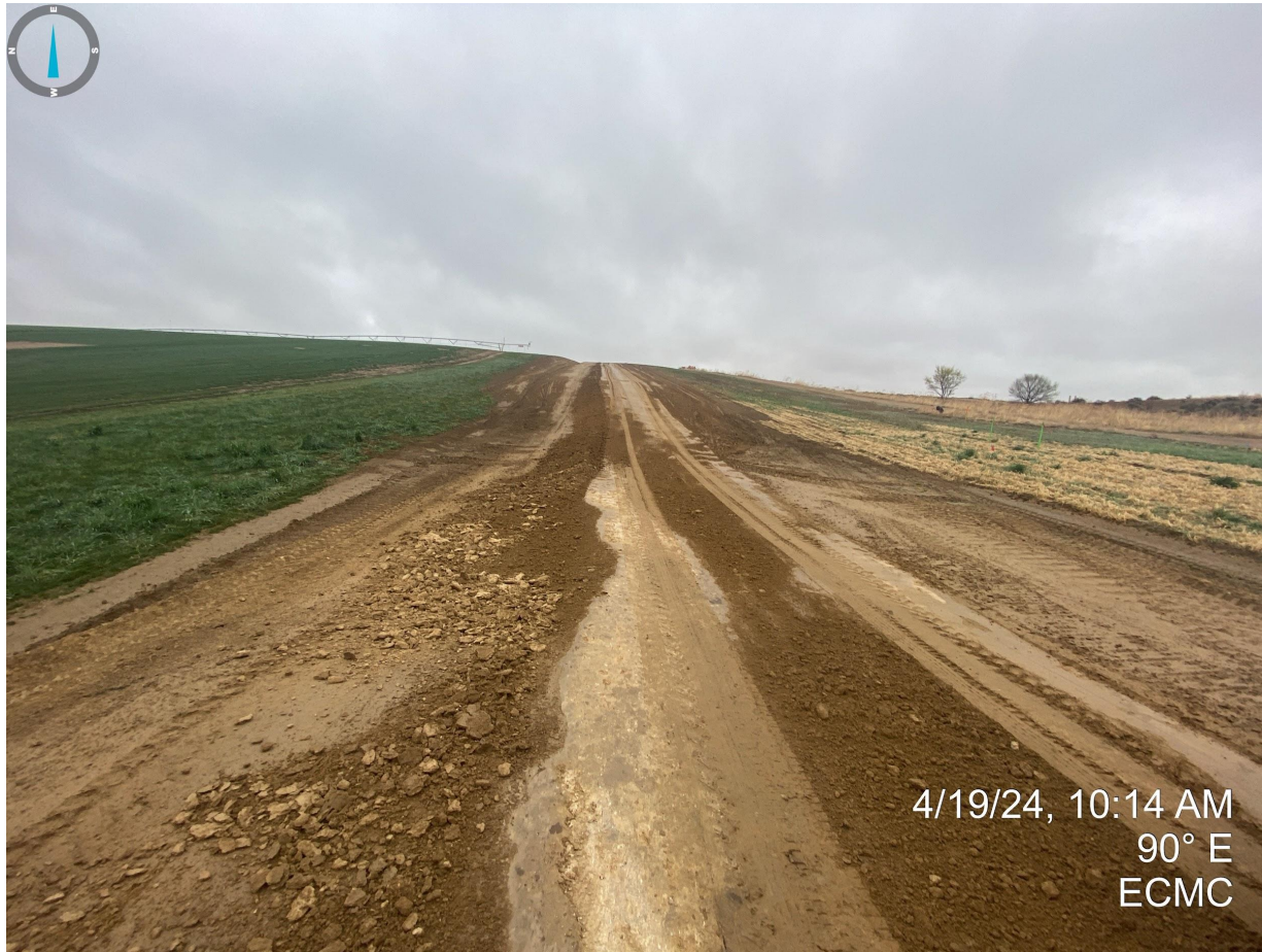
Photo 14. Taken near the center portion of the access road, facing east. See comments in Photo 12. It appears that stormwater BMPs are planned for the low point of the access road.
