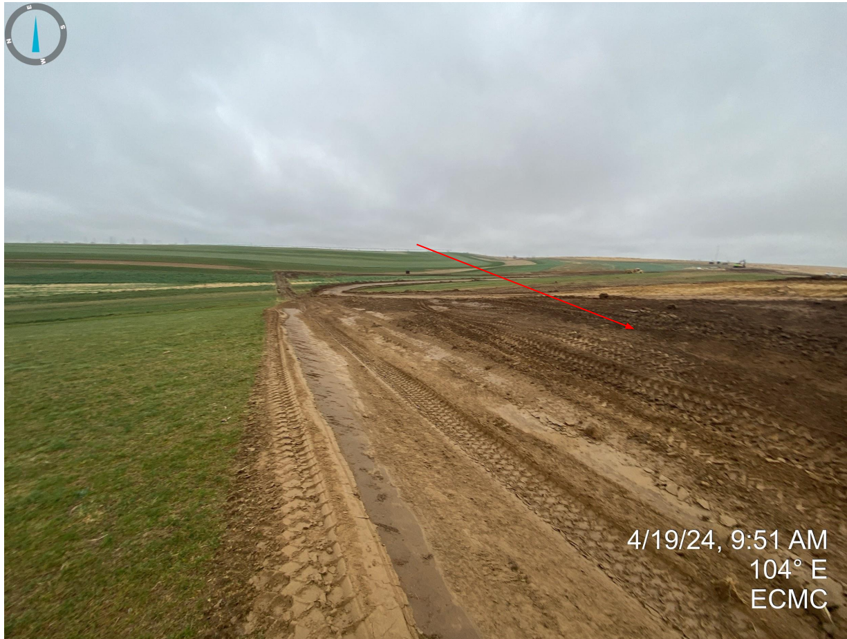
Photo 5. Stormwater ditch constructed along the north side of the disturbance area. Topsoil stockpile illustrated by red arrow.
