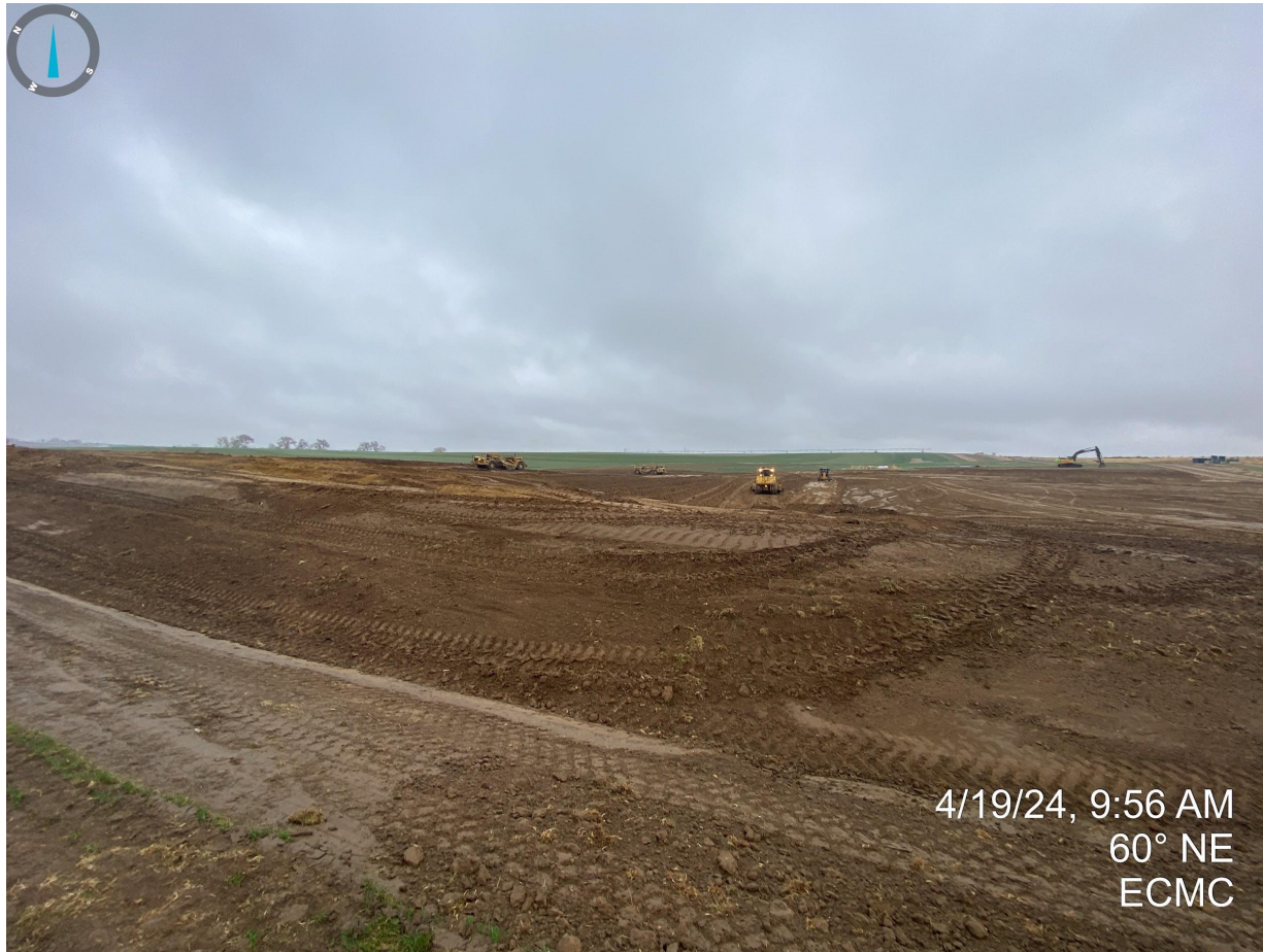
Photo 9. Taken near the west side of the disturbance area. Photo illustrates topsoil salvage activities and cut/fill operations are ongoing.
