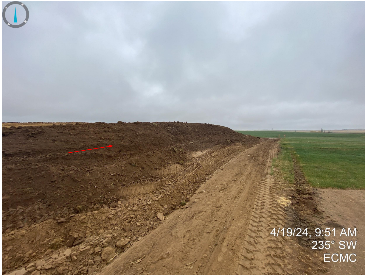
Photo 6. Stormwater ditch constructed along the north side of the disturbance area. Topsoil stockpile illustrated by red arrow.
