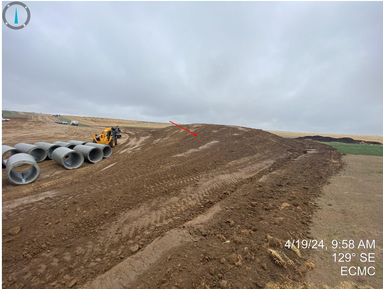
Photo 10. Topsoil stockpile located in the southwest corner of the disturbance area where the future production facility will be located. Operator shall ensure that all topsoil is stabilized in compliance with Rule 1002.c.
