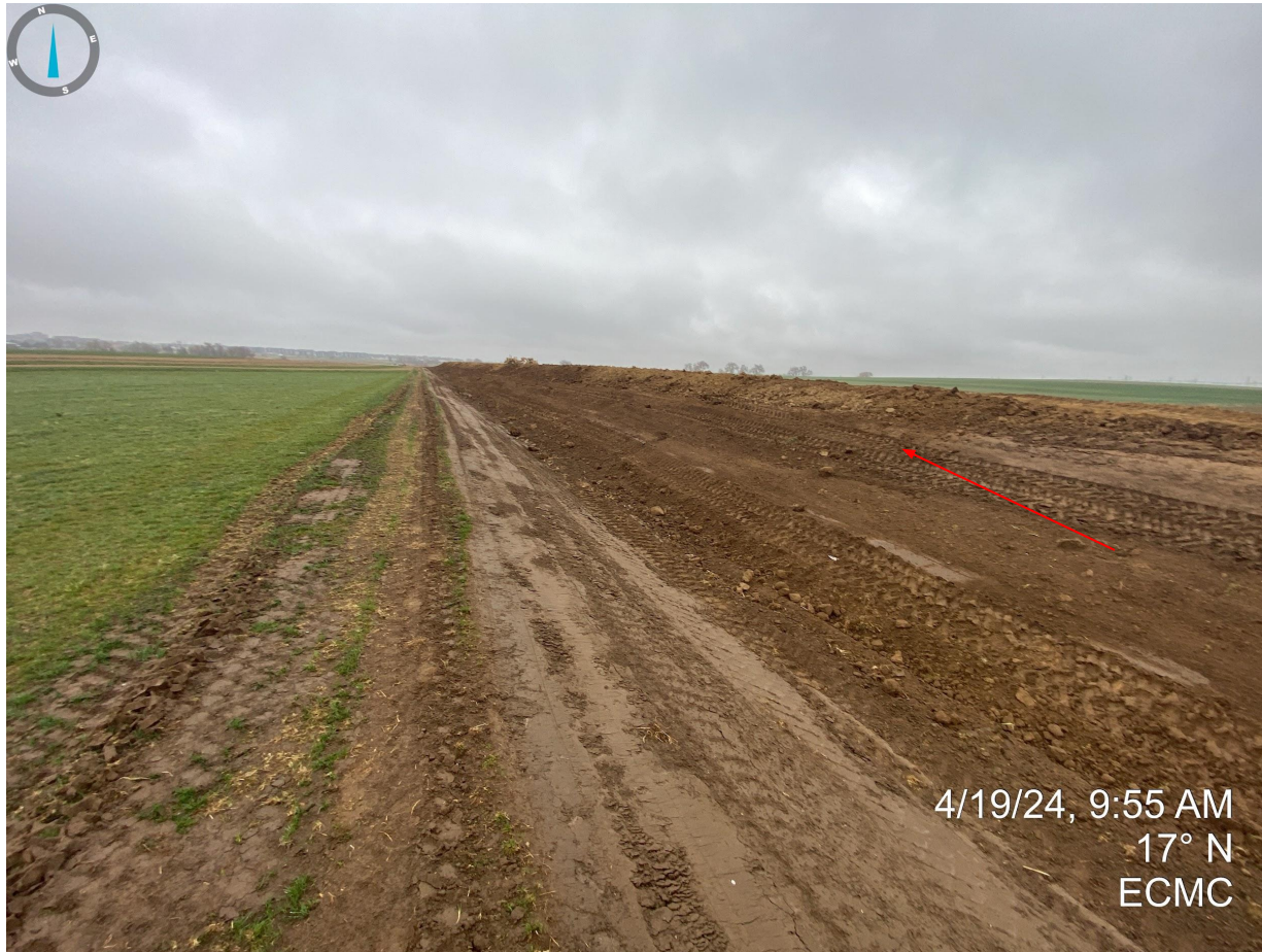
Photo 8. Stormwater ditch constructed along the west side of the disturbance area. Topsoil stockpile illustrated by red arrow.
