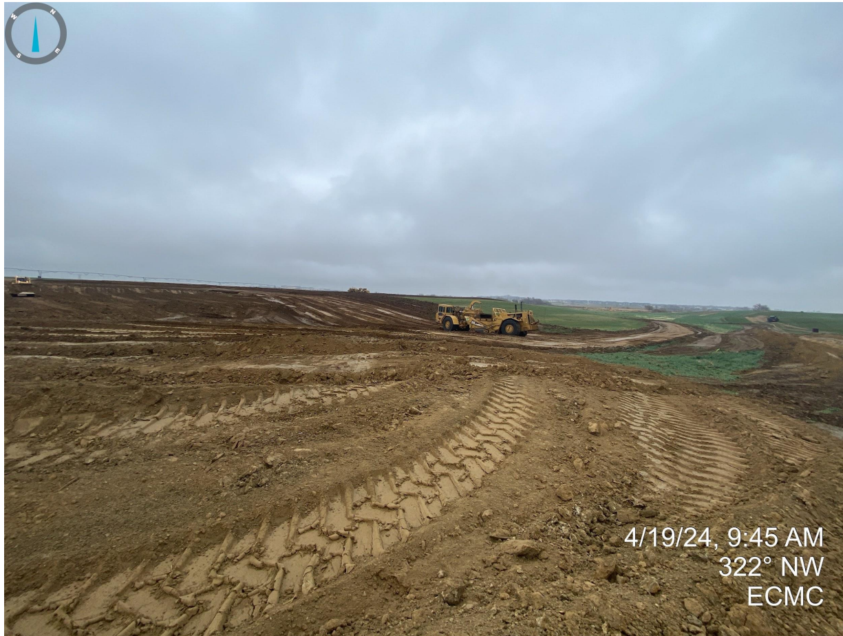
Photo 3. Taken near the east side of the disturbance area. Photo illustrates topsoil salvage activities and cut/fill operations.
