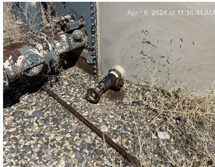
Stained soil from equipment leak
