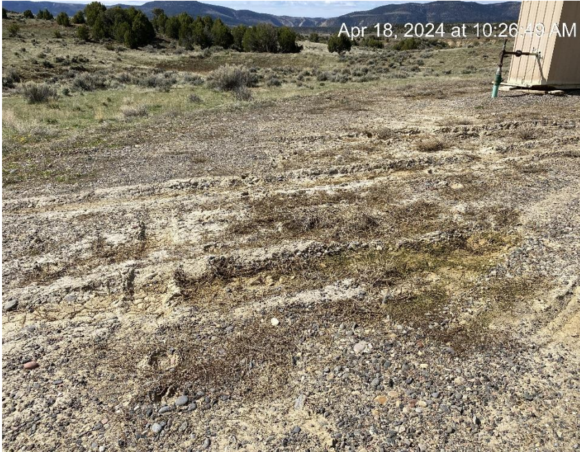
Erosion and sediment migration
