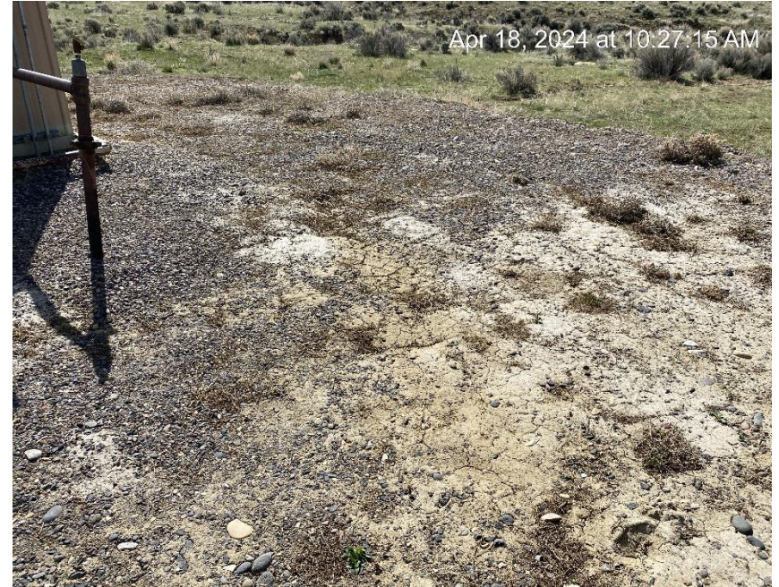
Erosion and sediment migration
