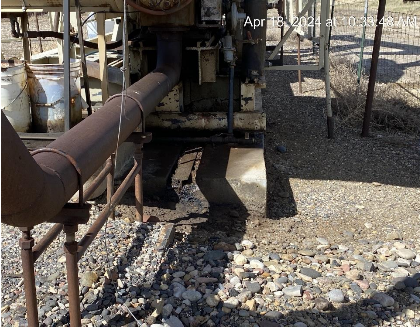
Equipment leaks. Stained soil.
