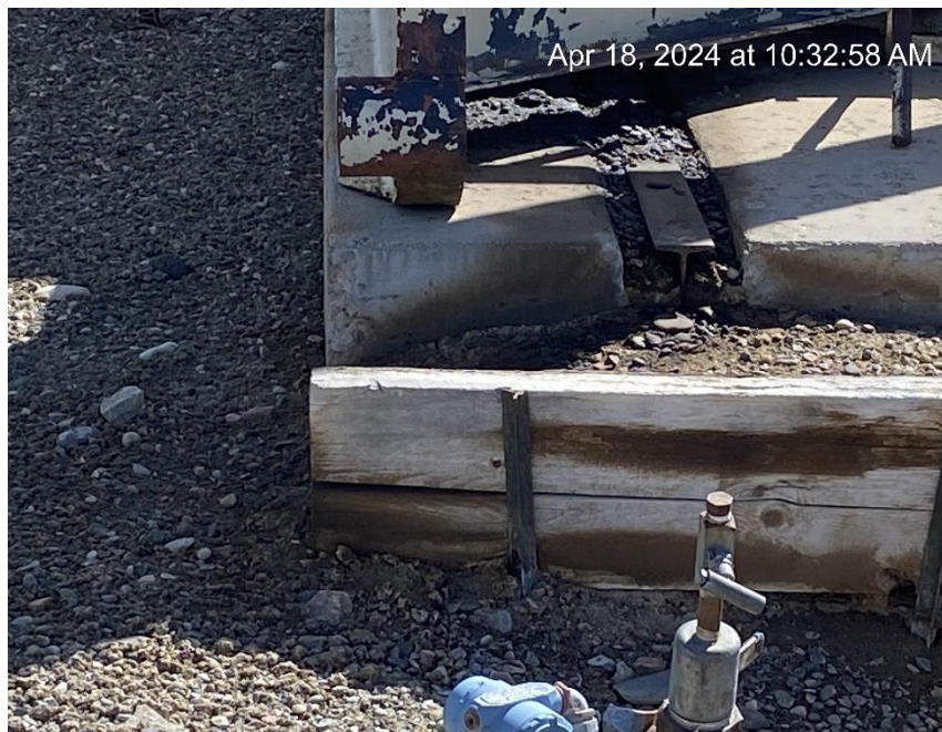
Equipment leak and stained soil
