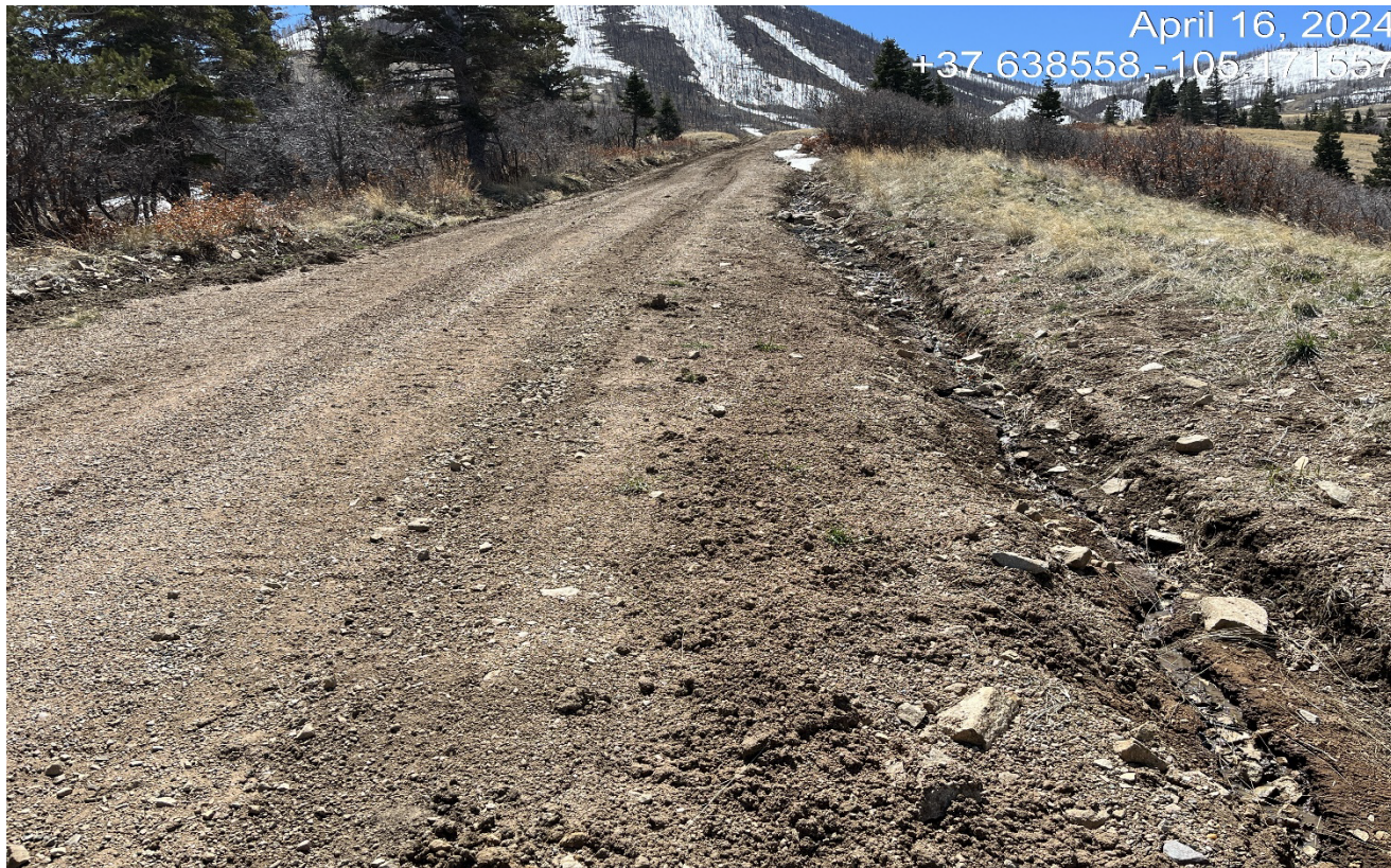
Photo 1. Facing south along the access road. There is erosion along the roadside that has not been repaired and BMP's have not been installed. Previous corrective action has not been completed.
