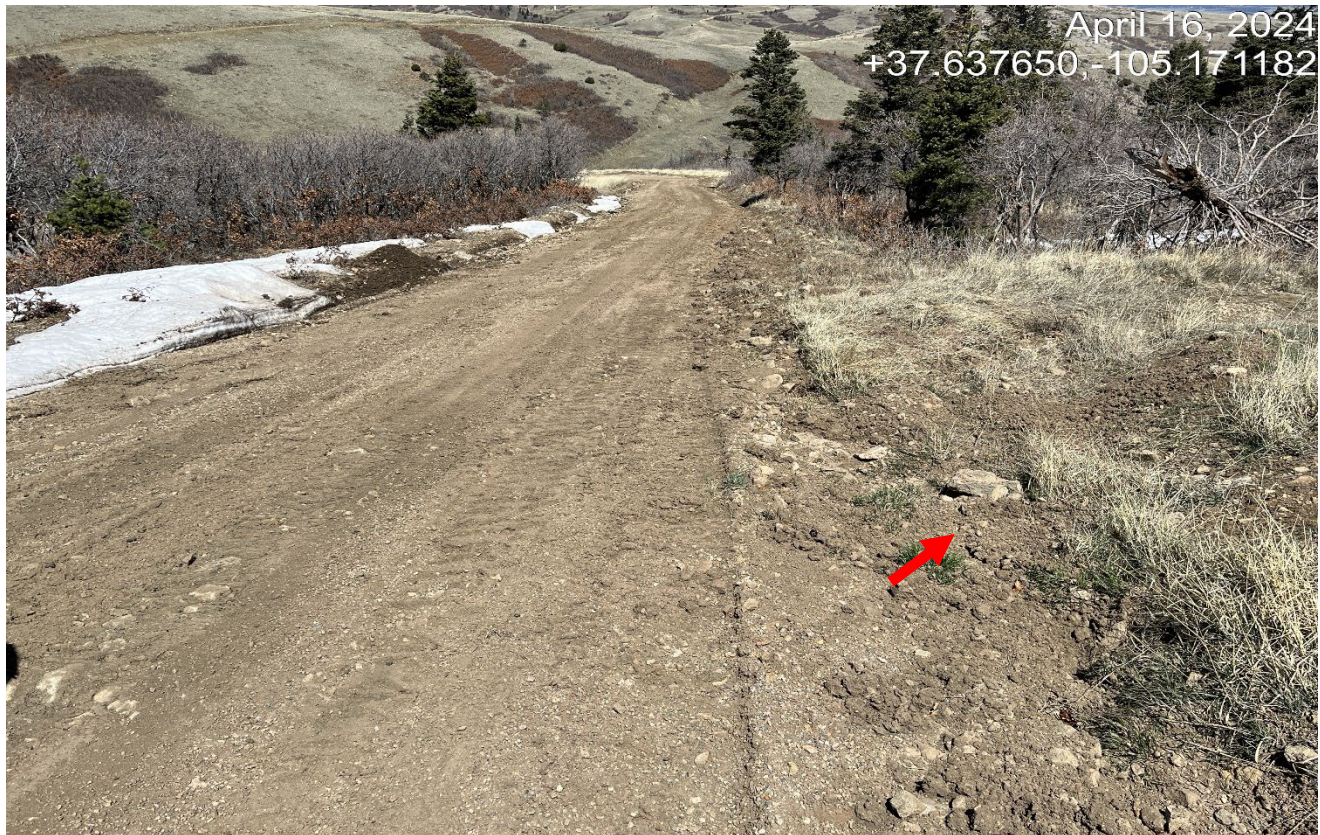
Photo 3. Facing back north the steep grade of access road. Stormwater is not being diverted off the road which is causing erosion of the road. Stormwater should be divert toward red arrow and into a sediment trap.
