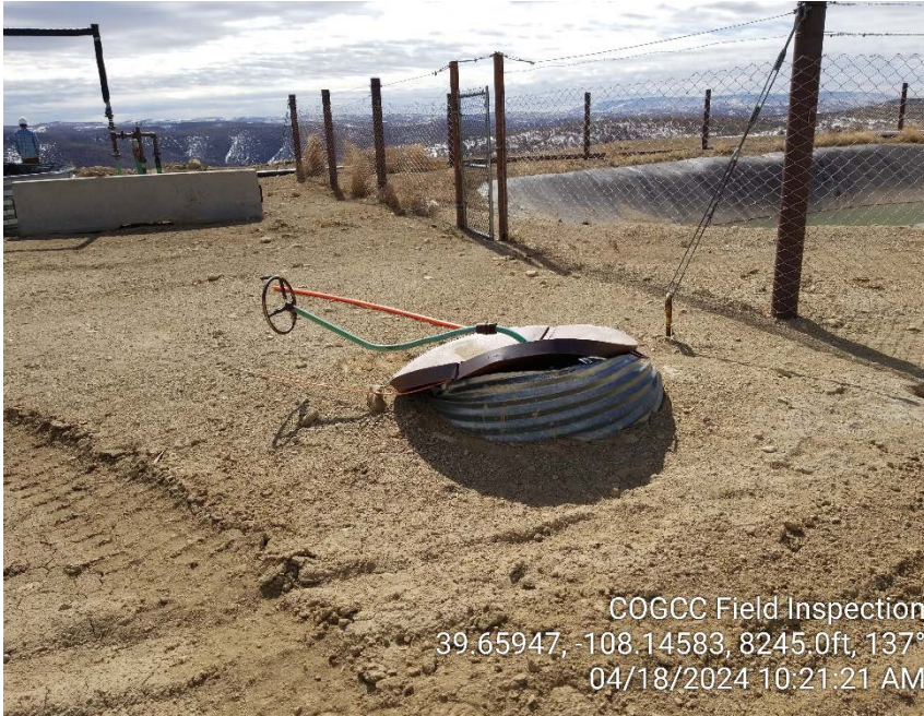
Photo #7 – Damaged valve can at NW corner of pit.
