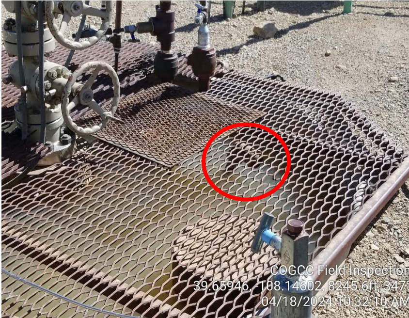
Photo #21 - Uncapped wellhead equipment in well cellar.
