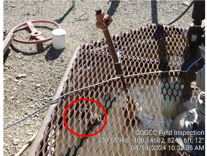
Photo #20 – Uncapped wellhead equipment in well cellar.
