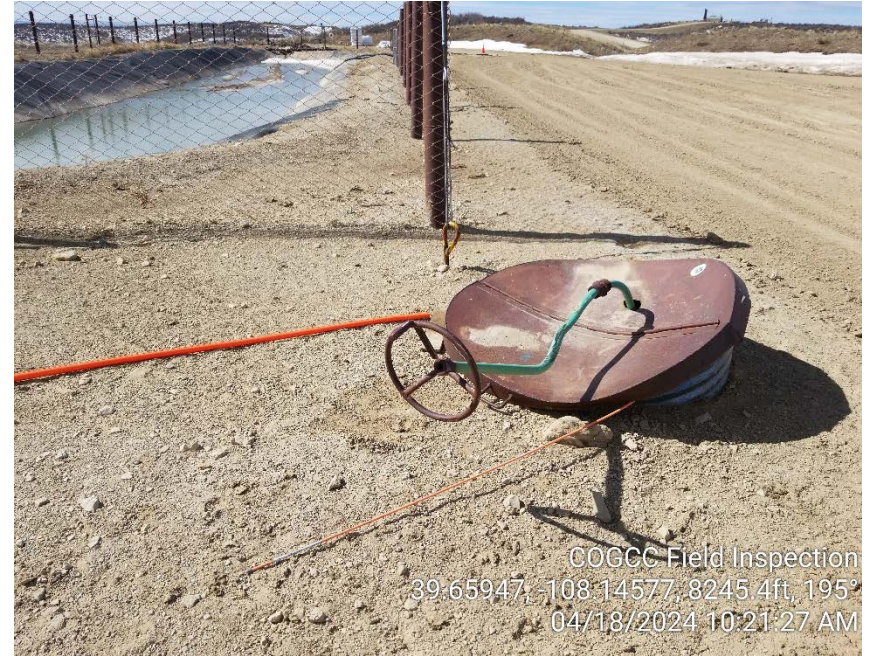
Photo #8 - Damaged valve can at NW corner of pit (2).
