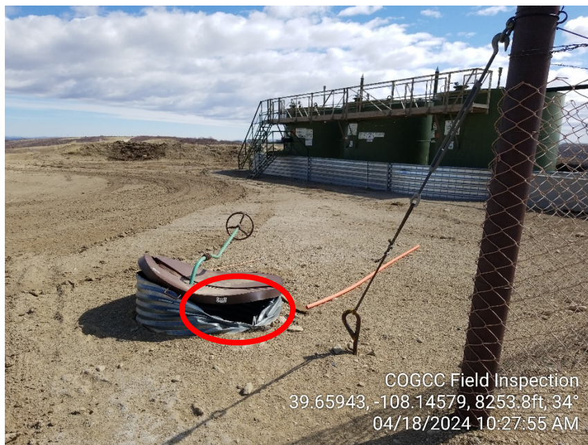
Photo #9 - Damaged valve can at NW corner of pit (3).
