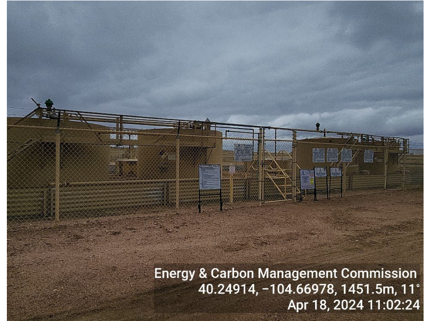
Photo 8: Centralized tank battery
