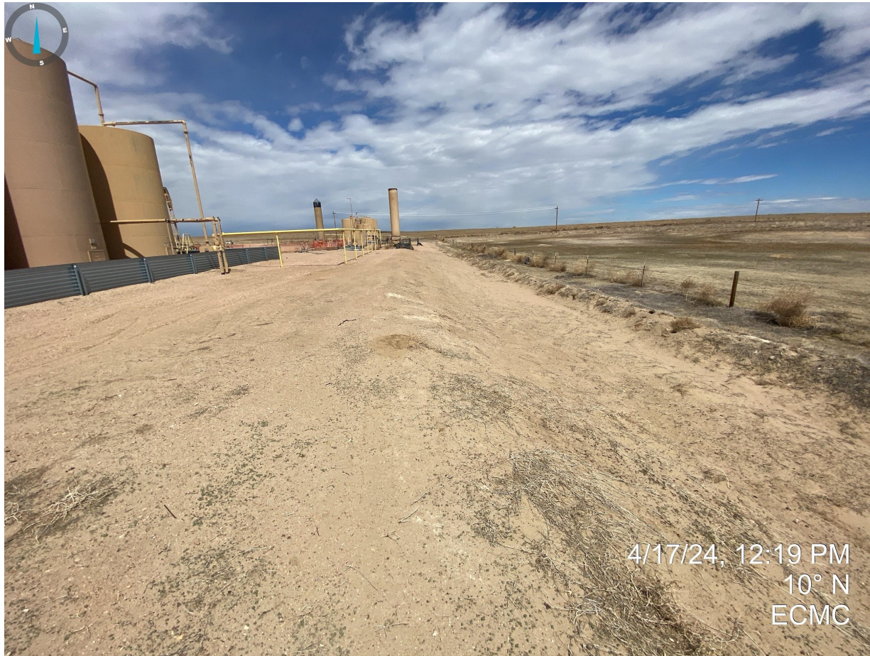
Photo 3. Production areas are not properly stabilized as they are primarily exposed soils.
