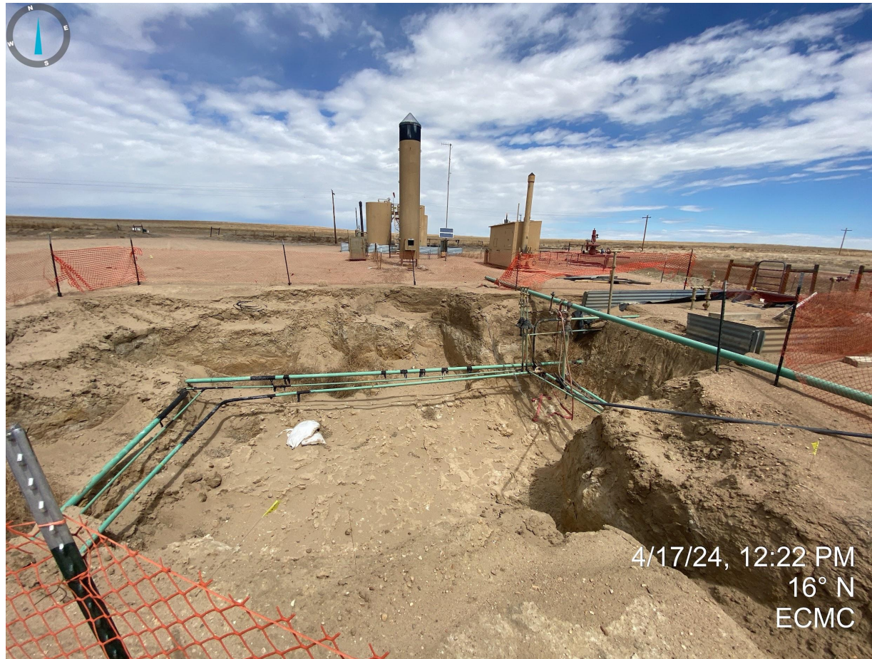
Photo 7. Open excavation in relation to remediation project #33589. Operator shall continue to follow 900 series rules for project closure and maintain fencing around all open excavations.
