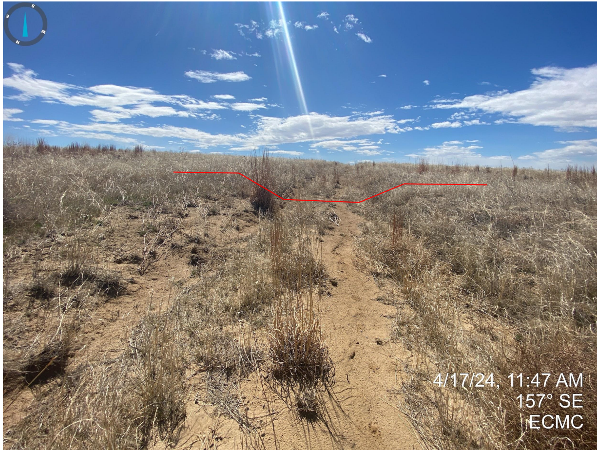
Photo 1. Access road has not been recontoured/graded to reflect adjacent topography.
