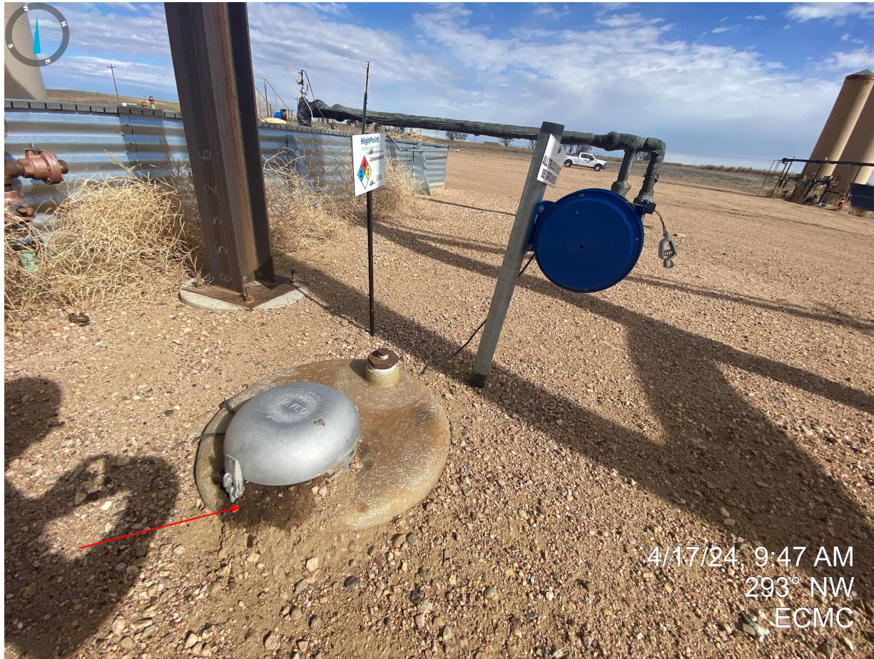
Photo 8. Stained soil around buried vessel needs to be cleaned up and properly disposed of.
