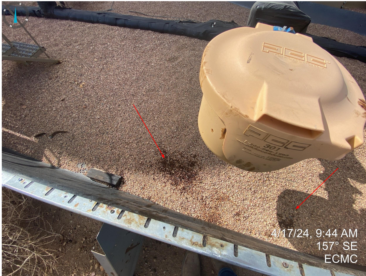
Photo 7. Stained soil within secondary containment needs to be properly cleaned up and removed.
