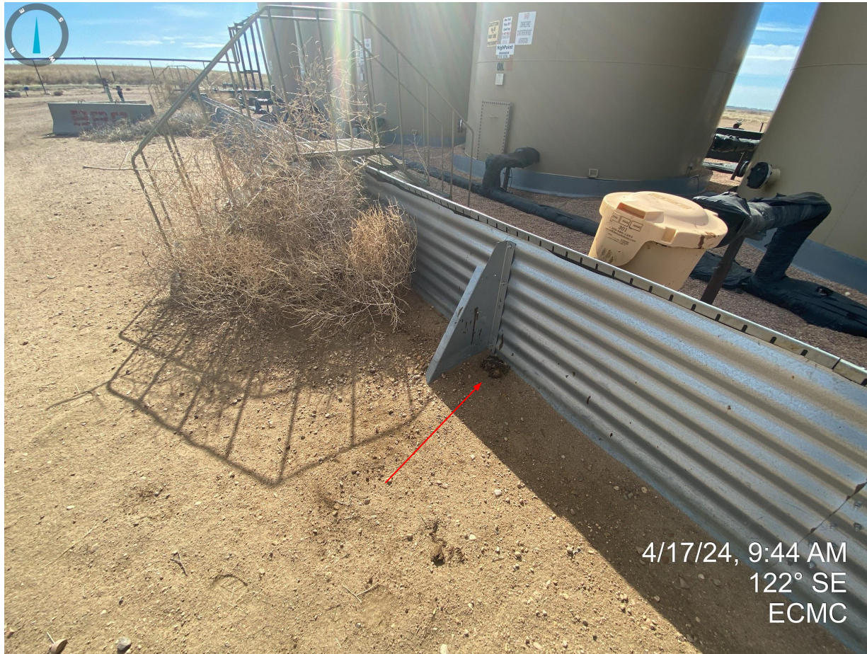
Photo 11. Stained soil outside of secondary equipment needs to be removed and properly disposed of.
