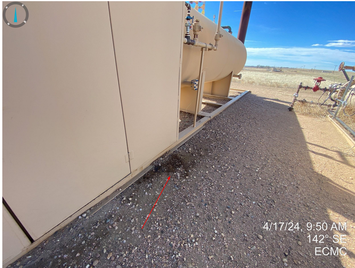
Photo 9. Stained soil around equipment needs to be properly cleaned up and disposed of.
