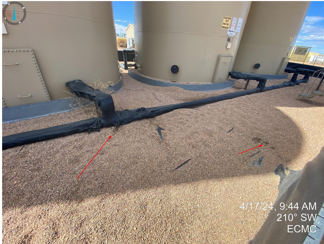
Photo 6. Stained soil within secondary containment needs to be properly cleaned up and removed.
