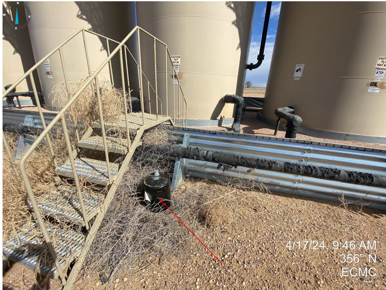
Photo 12. Container outside of secondary containment needs to be removed or placed inside of secondary containment.
