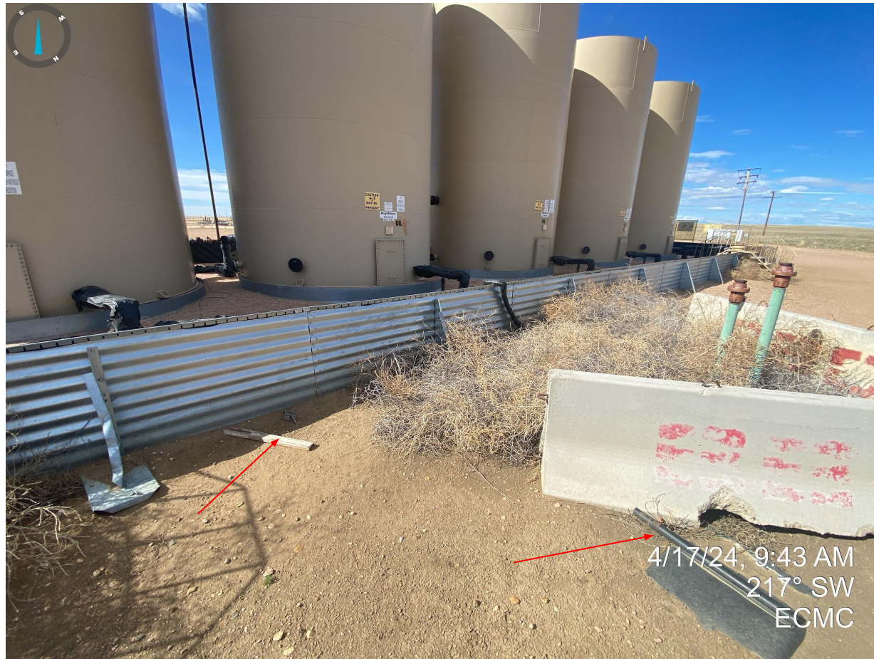
Photo 5. Tumbleweed accumulations and debris/trash need to be removed.
