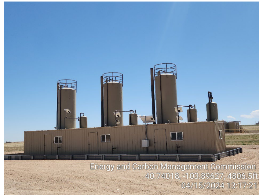
Photo 4 – Heater Treaters and Propane Tank
