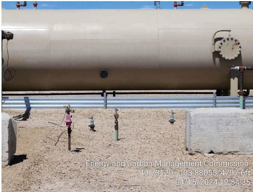
Photo 15 – Unmarked Risers at VRU
