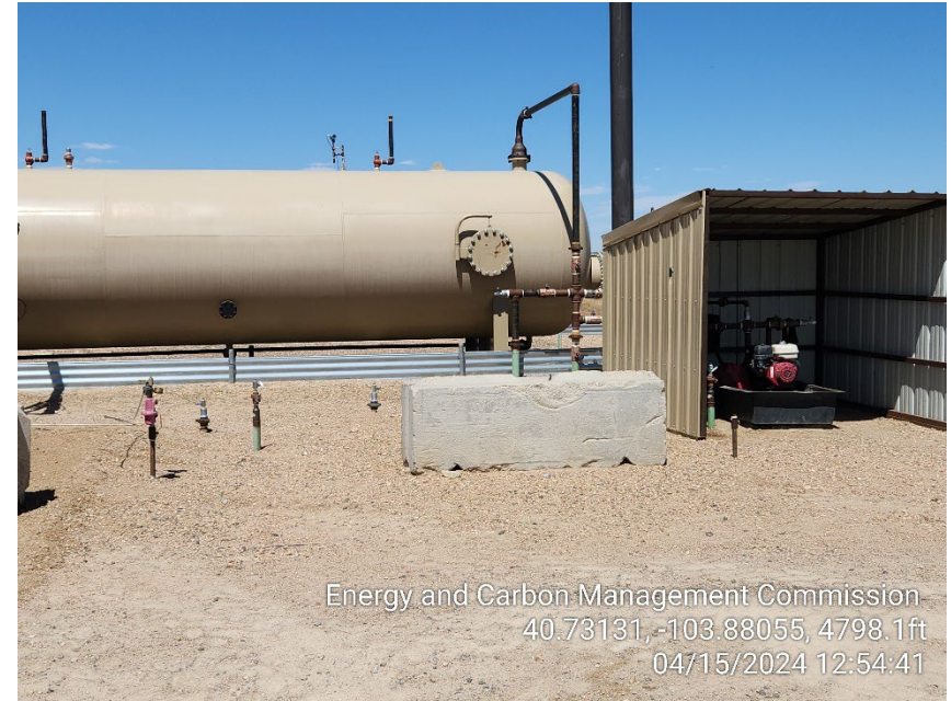
Photo 16 – Unmarked Risers at VRU
