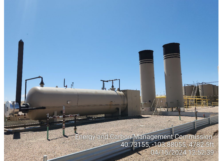
Photo 10 – Separator and ECDs
