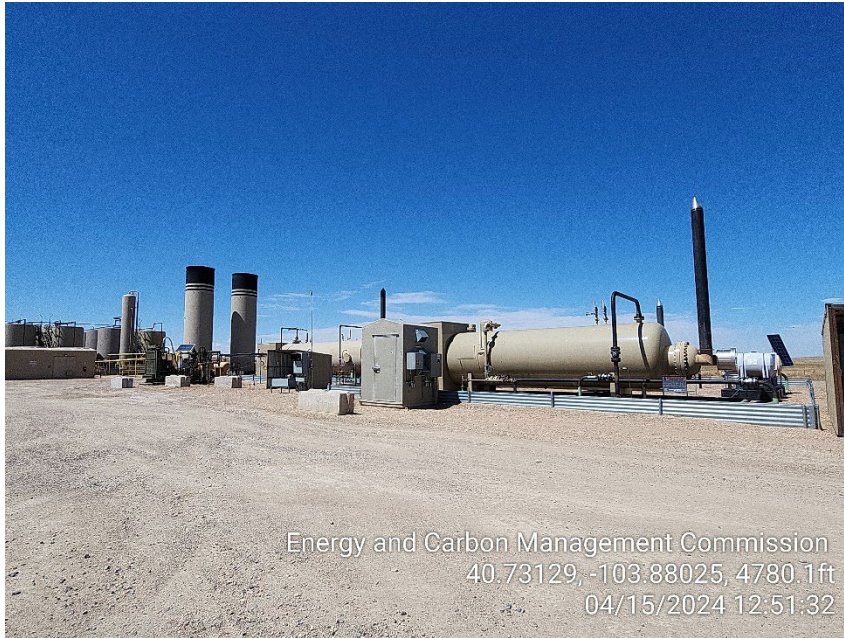
Photo 5 – Separator, Instrumental Air Unit and ECDs
