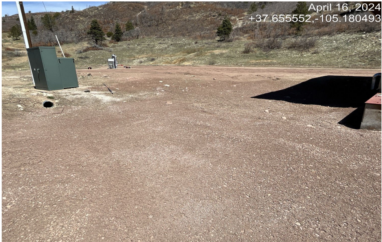
Photo 3. The remediation rea where tank was located has been backfilled with sand and gravel.
