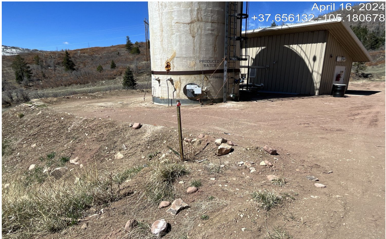
Photo 1. Facing toward the produced water tank. The secondary berm around the tank is insufficient to contain a spill. Red arrow points to small berm which could easily be overtopped by a leak. Previous corrective action was not completed.
