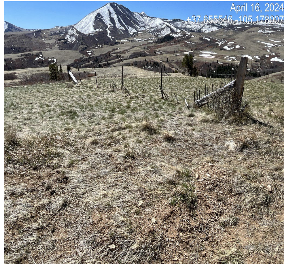
Photo 12. Observed along the access road were several dilapidated snow fences which need to be removed or repaired. Previous corrective action was not completed.
