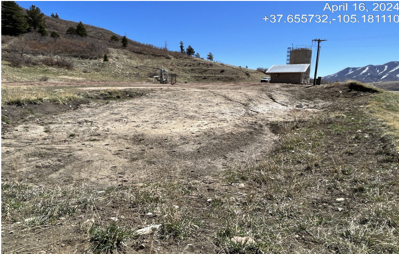
Photo 6. Facing southeast at the down gradient portion of the location. The degraded perimeter wattles were removed however, no new BMP's were installed and there is a creek approximately 10ft' from the edge of the location. Previous corrective action has not been completed.
