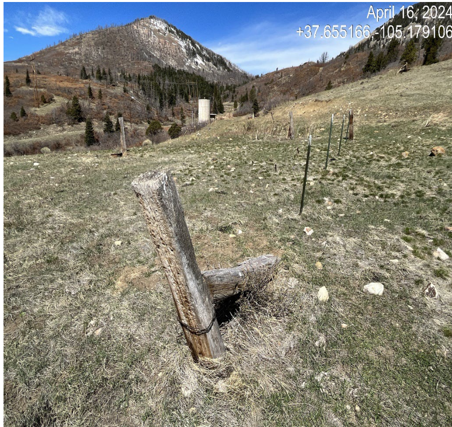
Photo 12. Observed along the access road were several dilapidated snow fences which need to be removed or repaired. Previous corrective action was not completed.
