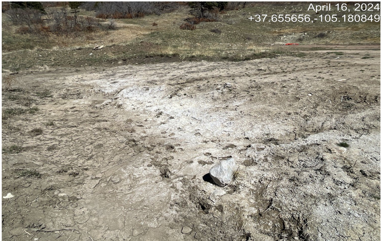
Photo 5. There is a white material used to backfill the excavated retention pond area and there are concerns this material may not be suitable for reclamation. Operator will need to sample this area for soil suitability.
