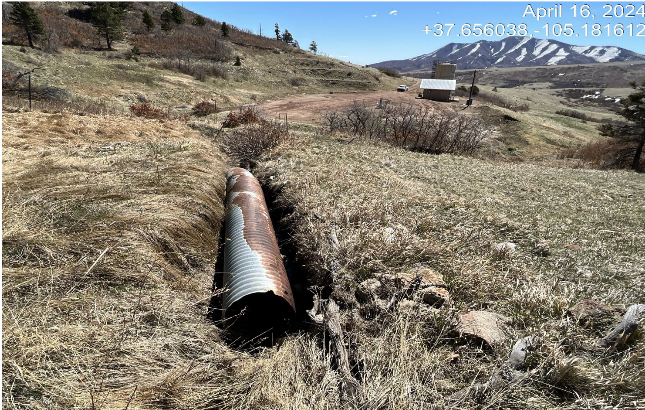
Photo 9. Standing approximately 125' northwest of the location along the flowline area is an eroded out culvert where the creek flows. The culvert needs repaired or removed. Previous corrective action was not completed.
