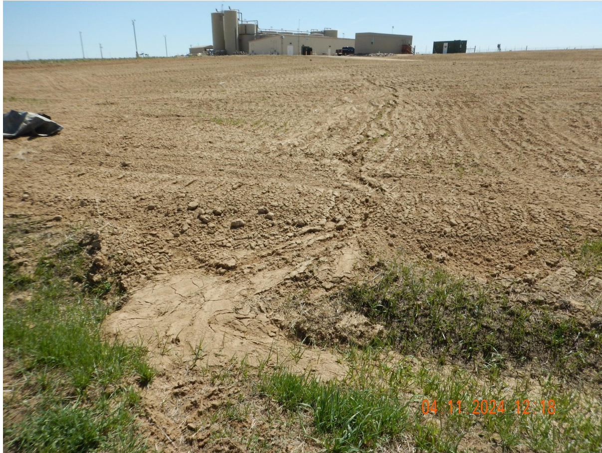
Photo 6. Photo taken from the northern interim reclamation area, facing South. Photo illustrates Operator has not properly tracked the fill slope, which is only aiding stormwater erosion towards an irrigation ditch.
