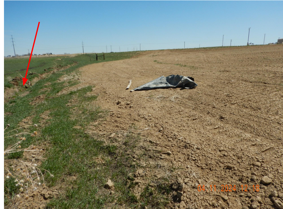
Photo 5. Photo taken from the northern interim reclamation area, facing East. Photo illustrates there is no perimeter stormwater BMP, only a remnant insufficient ditch area along small portions of the perimeter. Red arrow illustrates the irrigation ditch.
