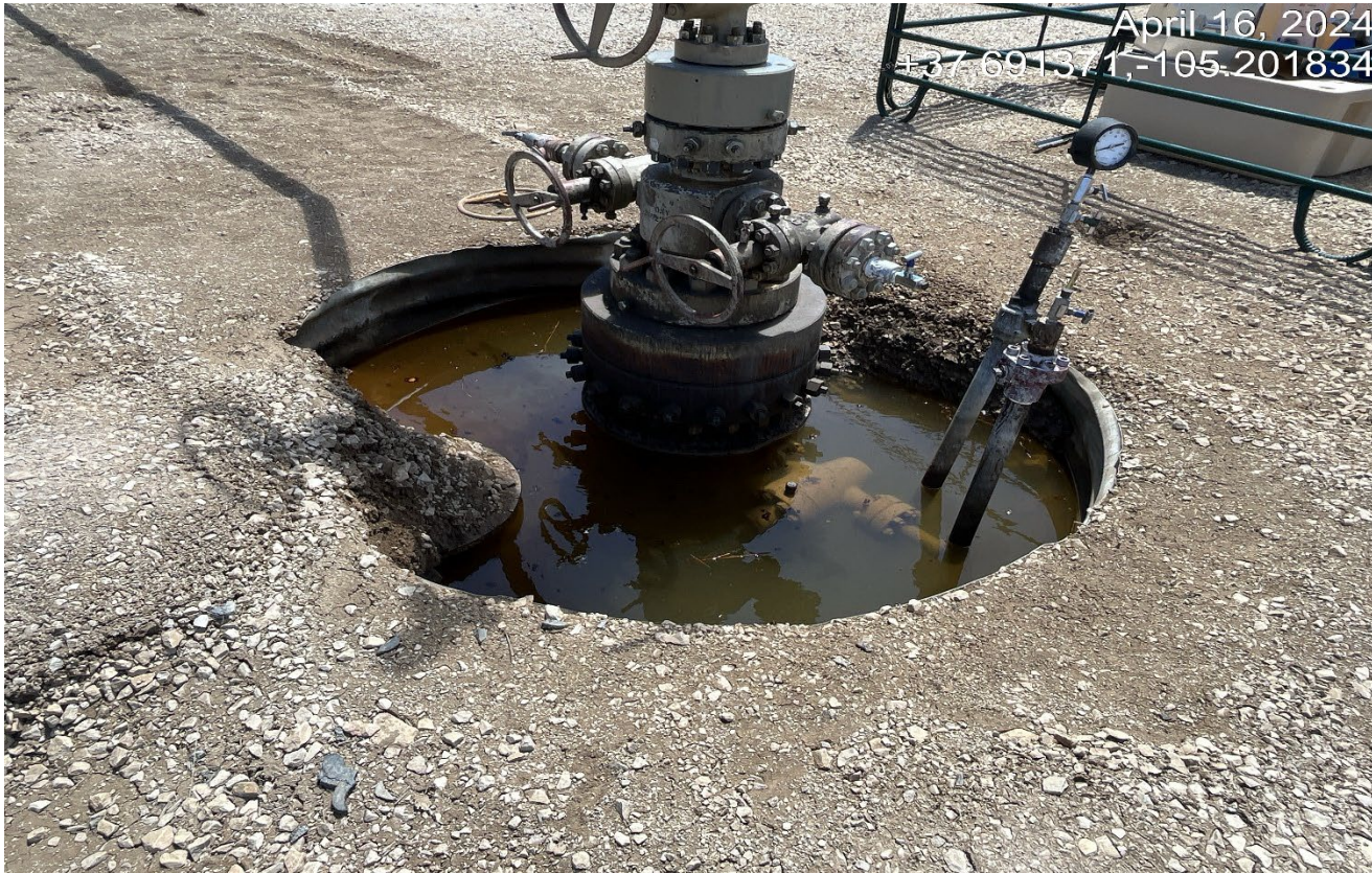
Photo 2. There is an oily sheen in the water at the well cellar.
