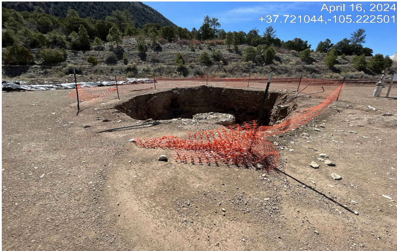
Photo 9. Facing toward the open excavation which the fence has fall apart. This must be fenced immediately to prevent wildlife of livestock from falling in.
