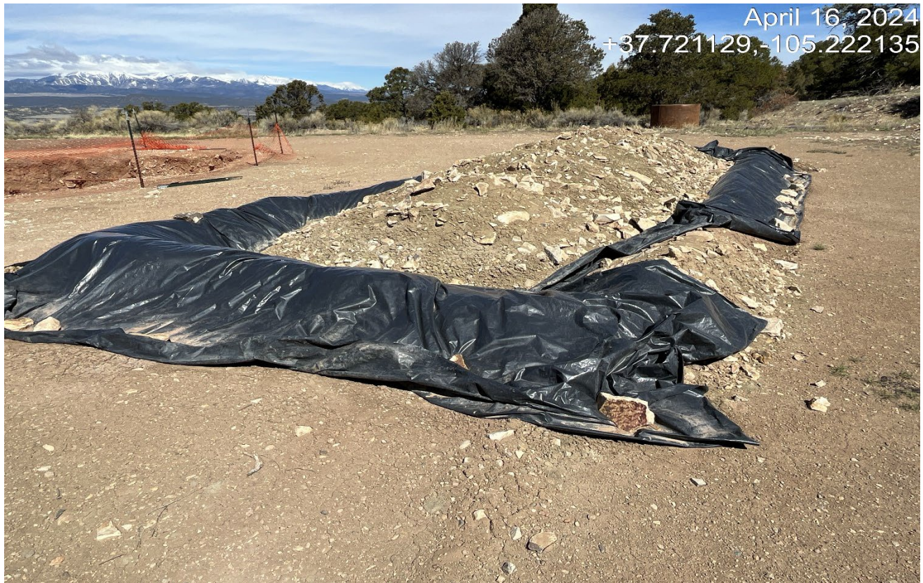
Photo 10. The plastic liner is compromised and impacted soil needs to be removed.
