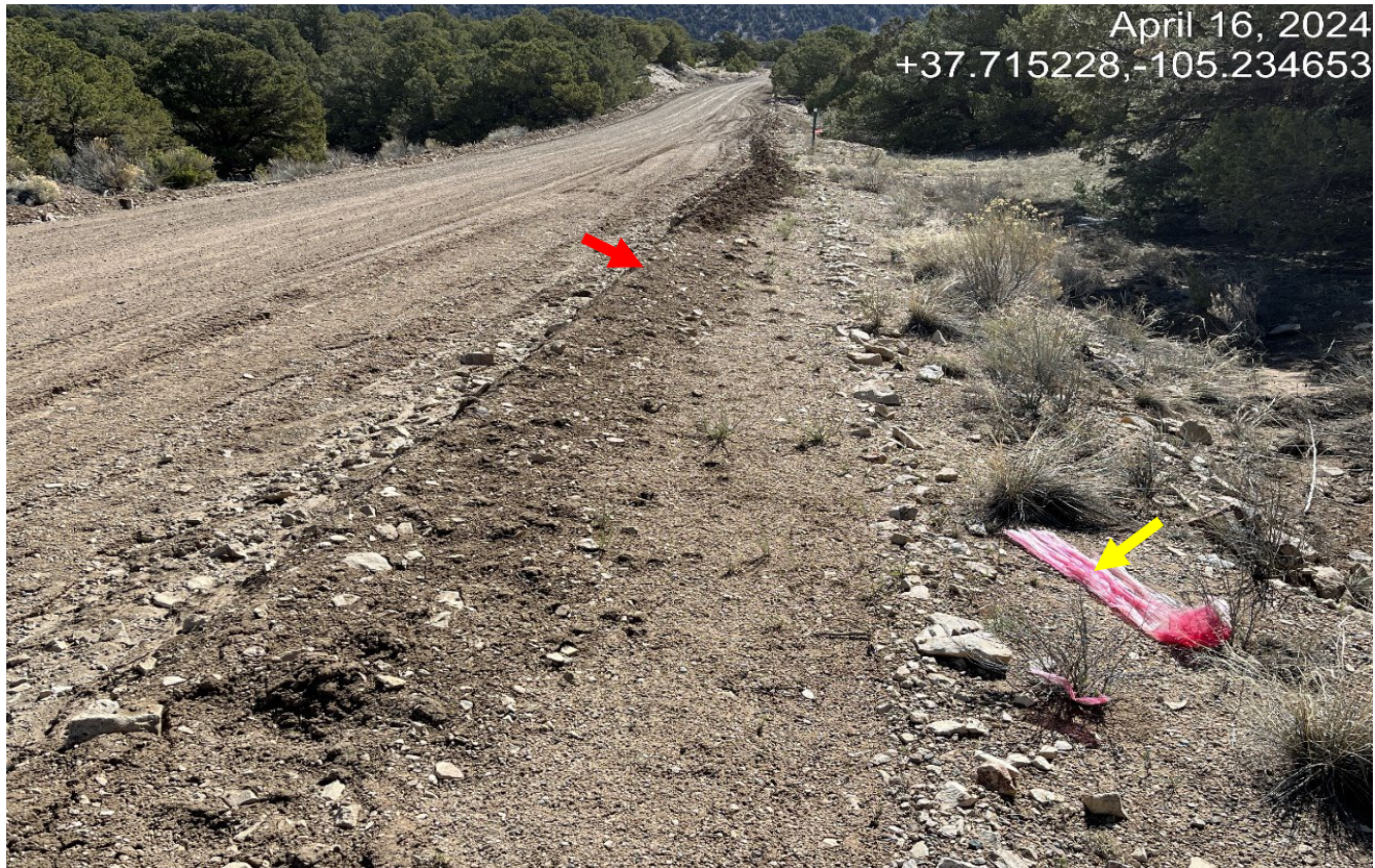
Photo 3. Facing east along the access road. Grading of the road has pushed a row of gravel along the side shown at red arrow which interferes which stormwater drainage off the road to prevent erosion. There is trash at yellow arrow that needs to be pick up.
