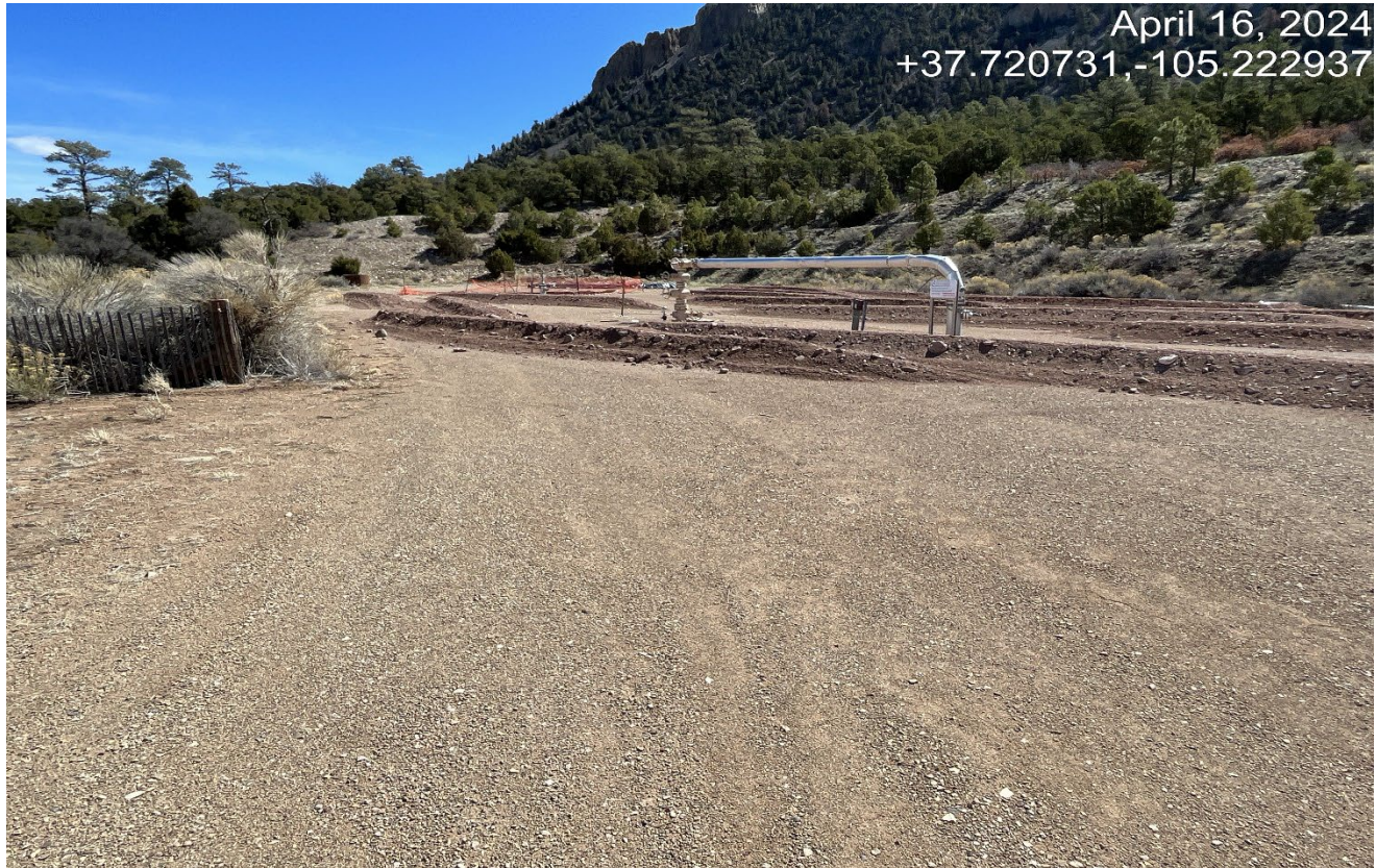
Photo 7. Facing northeast toward the wellsite. Fill material has been brought in to backfill the open excavation..
