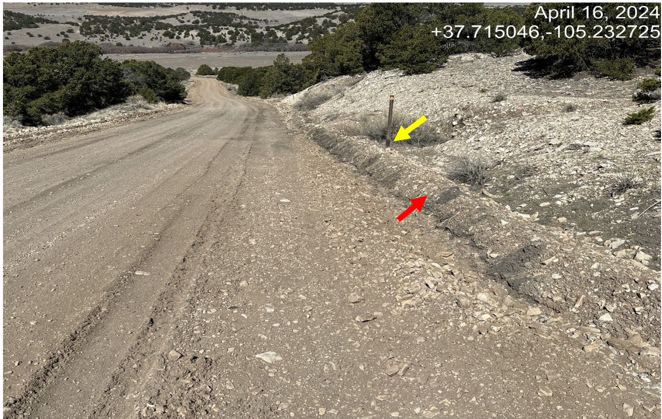
Photo 4. Facing back west down the access road. Grading of the road has pushed a row of gravel along the side shown at red arrow which is blocking drainage toward the culvert at the yellow arrow.
