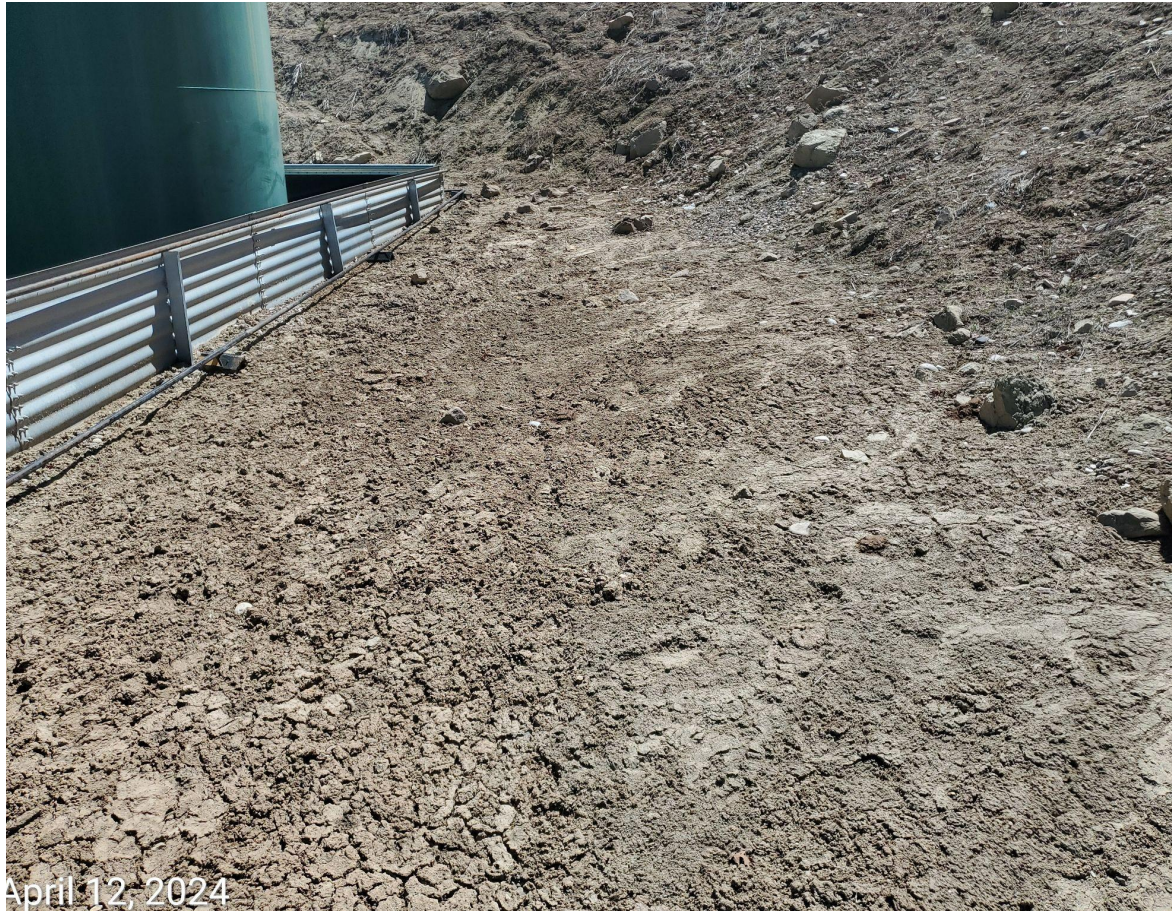
Photo 4: Continued from photo 3. Photo shows sediment deposition due to unstabilized slopes on the southern interim areas.
