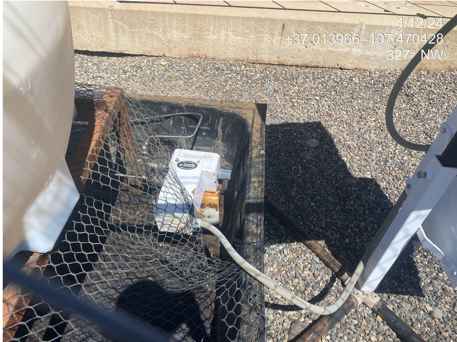
Photo 4. Wildlife netting covering plastic secondary containment at pump jack is no longer functioning, maintenance is required.
