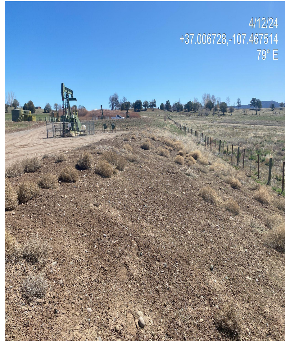
Photo 2. View of southern fill slope/interim reclamation areas dominated by kochia/russian thistle debris and lacking vegetation. Stormwater BMPs/soil stabilization is needed until long term stabilization is achieved with perennial vegetation.
