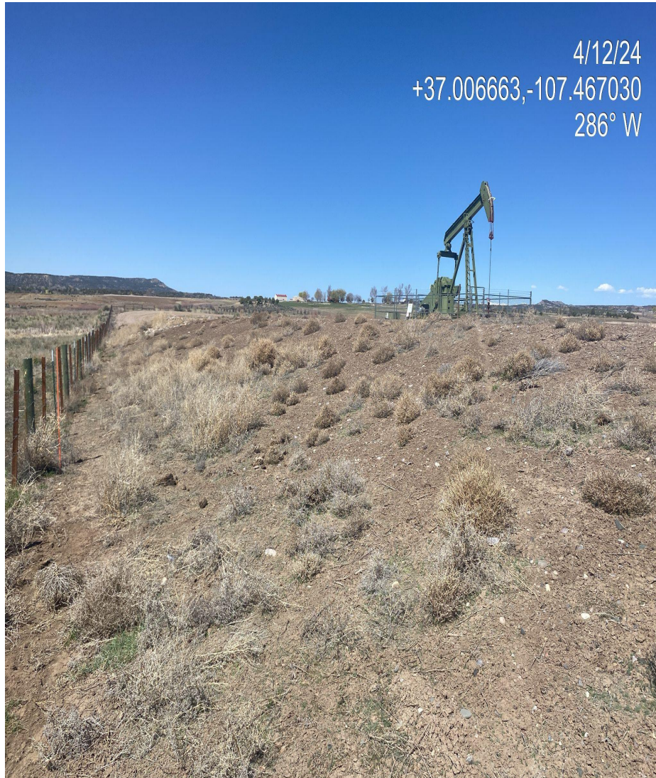
Photo 2. View of southern fill slope/interim reclamation areas dominated by kochia/russian thistle debris and lacking vegetation. Stormwater BMPs/soil stabilization is needed until long term stabilization is achieved with perennial vegetation.
