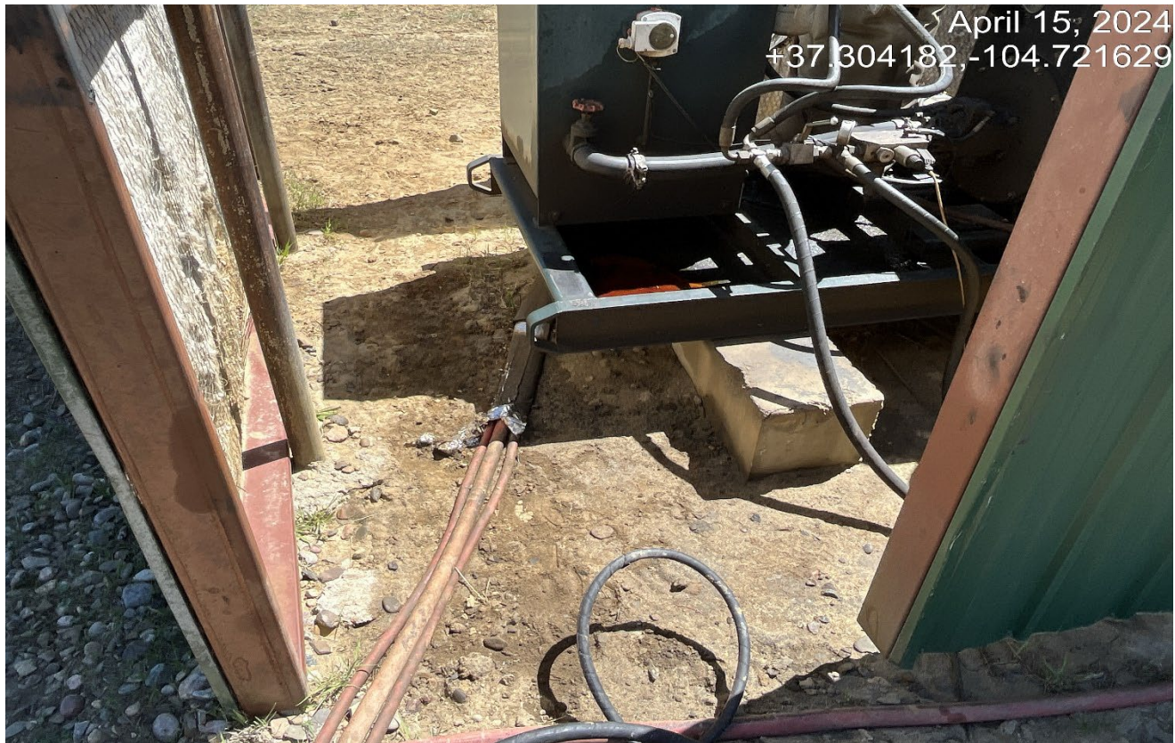
Photo 4. There is still oil stained soil by the engine skid and oil in the skid that needs to be cleaned up better.
