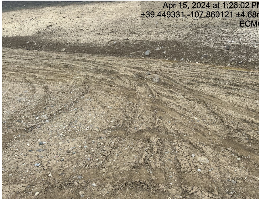
Areas of lack of stabilization/compaction
