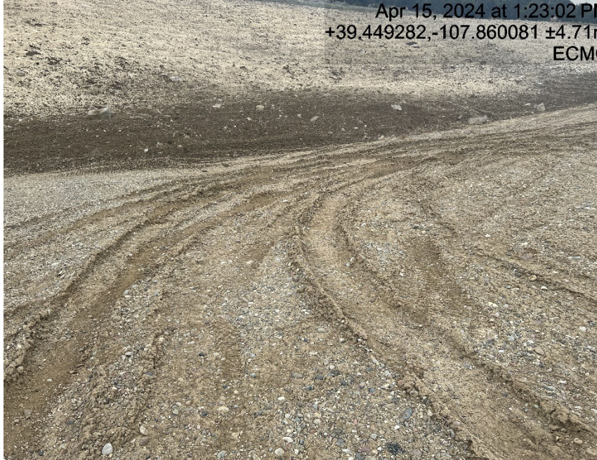
Areas of lack of stabilization/compaction
