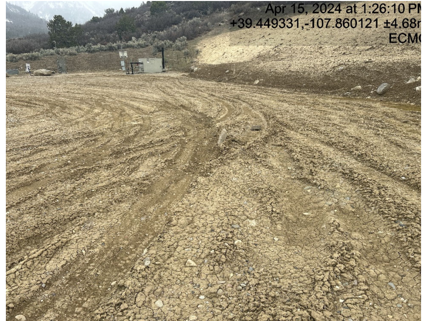
Areas of lack of stabilization/compaction
