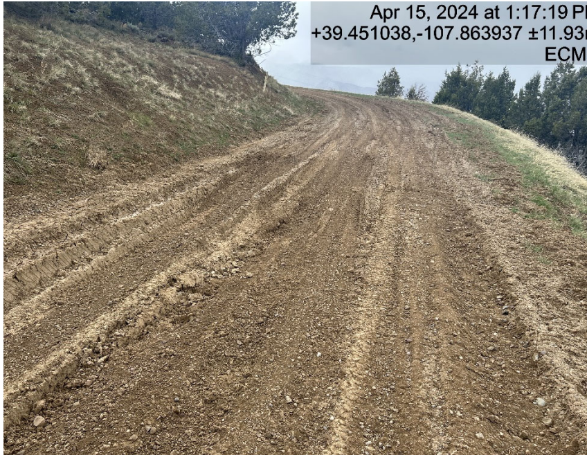
Areas of lack of stabilization/compaction
