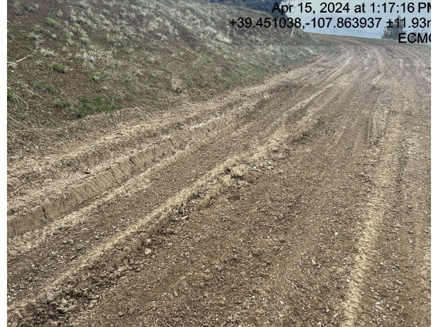
Areas of lack of stabilization/compaction
