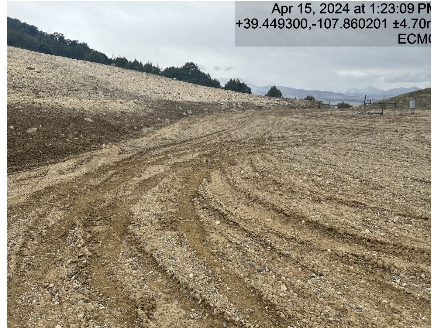
Areas of lack of stabilization/compaction
