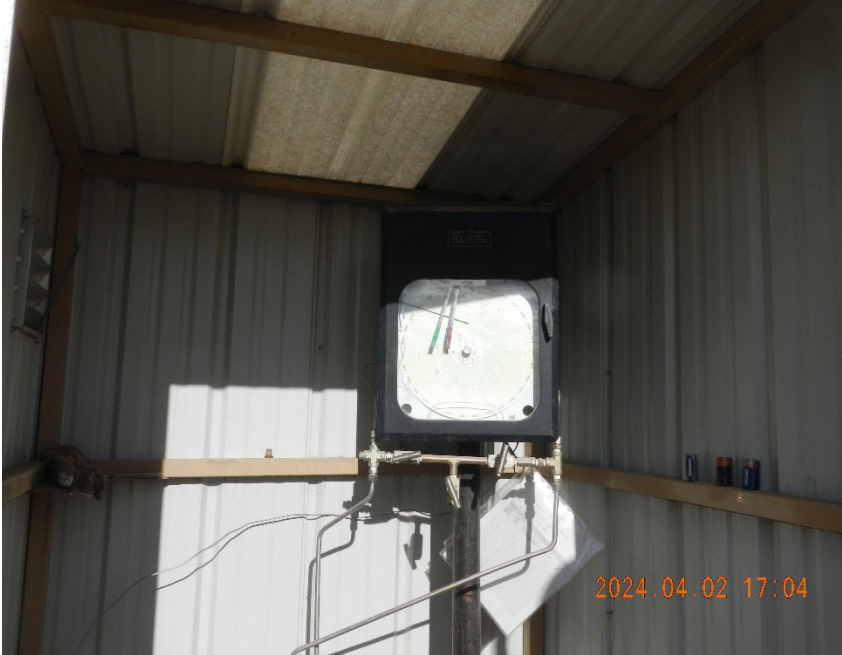
5. Gas meter inside meter shed.
