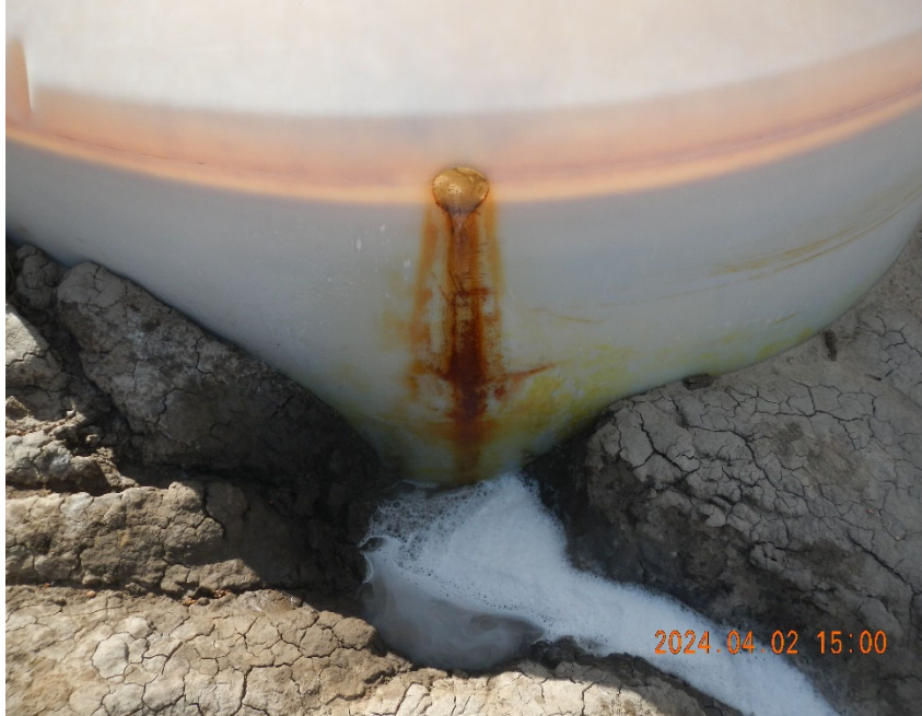
9. Produced water flowing out of side of tank wall. Line has been broken off or removed.
