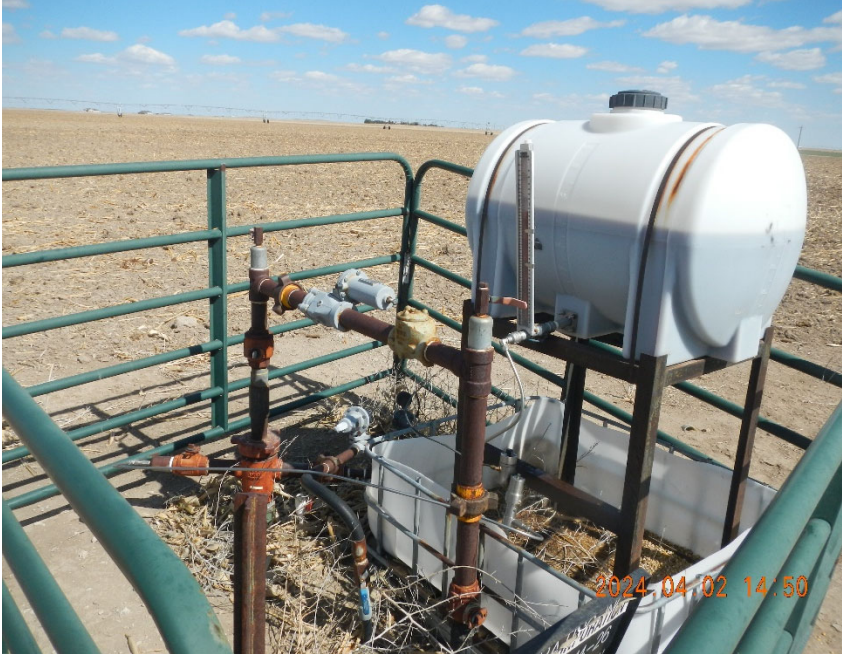
3. Chemical tank on secondary containment.
