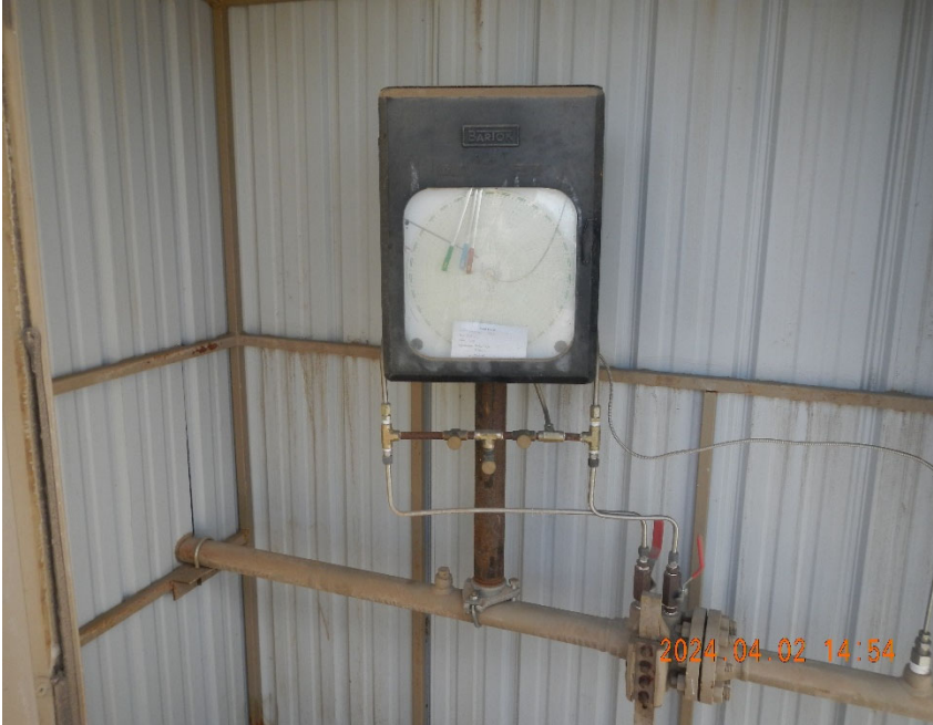
7. Gas meter inside meter shed.
