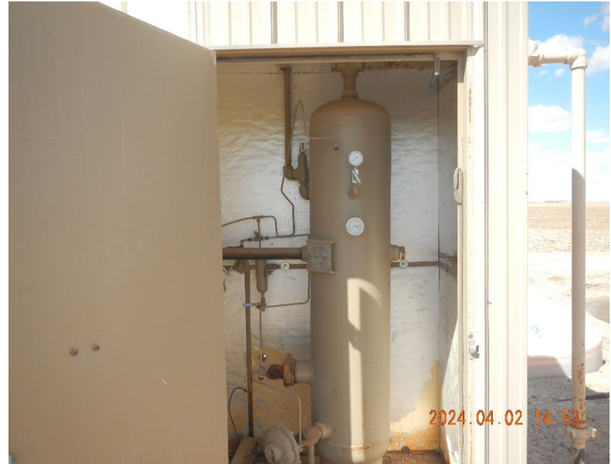
6. Vertical separator inside separator shed.
