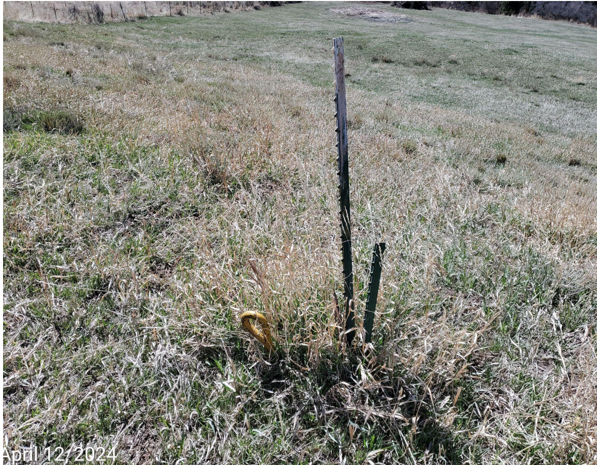
Photo 7: Photo example showing anchor equipment remaining. Equipment requires removal.
