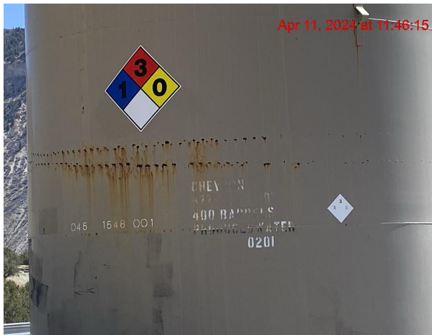
Painted Label for Tank Content/Capacity/Operator Contact Info is Weathered – Photo #00560
