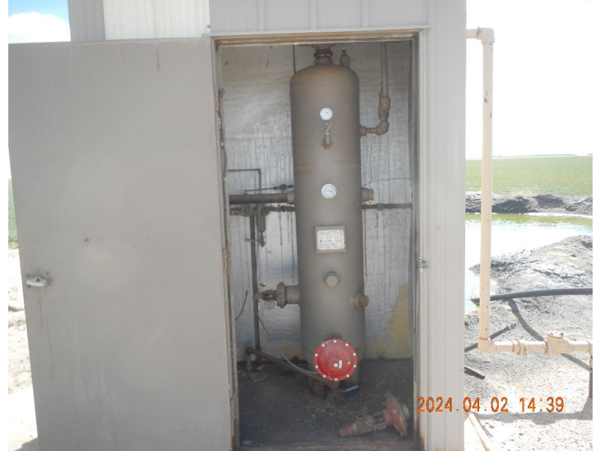
6. Vertical separator inside separator shed.
