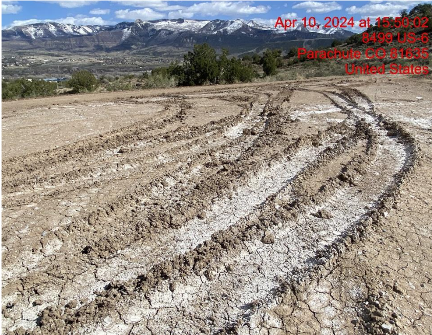
Lack of Stabilization/Insufficient Vehicle Tracking BMPs at Location Entrance/Exit – Photo #00533
