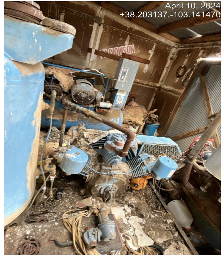
Photo 6&7. View of inside the shed shows debris and unmaintained equipment and supplies which is a fire hazard.
