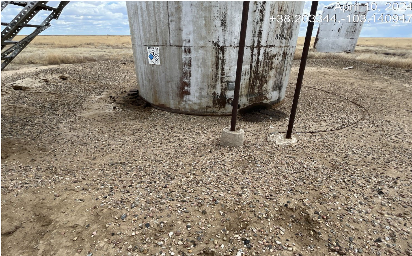
Photo 20. There is oily sludge at the base of the tank that needs to be cleaned up and properly disposed.
