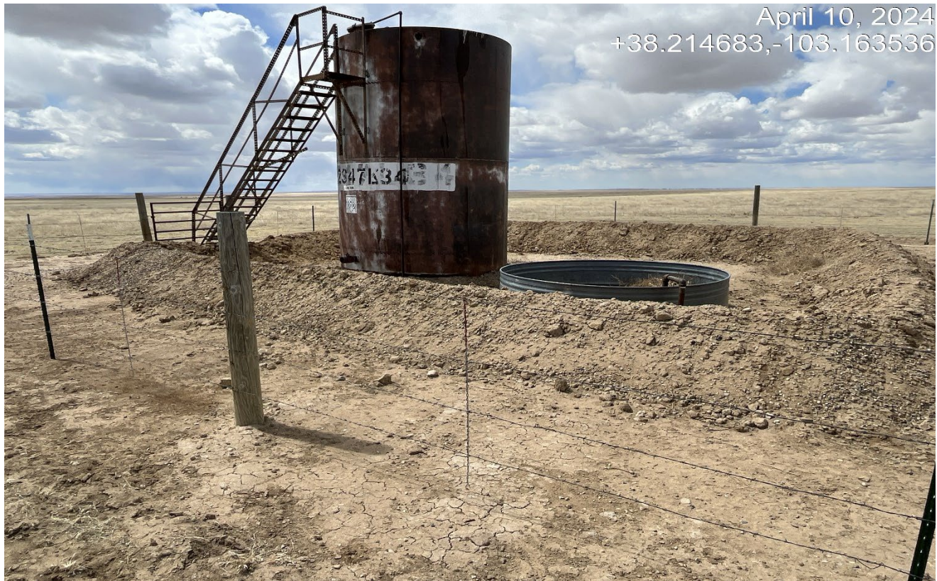
Photo 3. Facing toward the onsite tank which is fenced and a sufficient berm is constructed.
