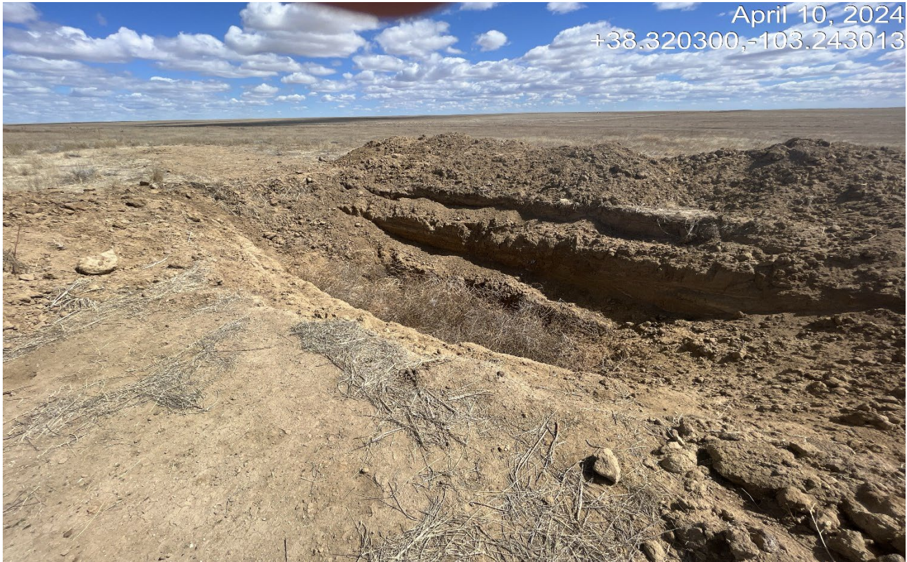
Photo 2. The well has been cut and capped below grade and open excavation remains.
