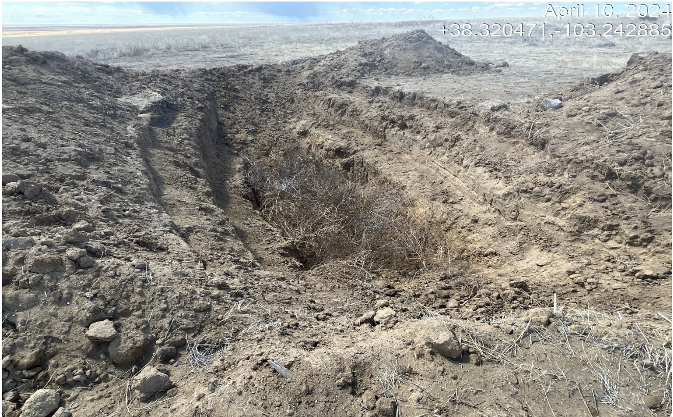
Photo 4. The open excavation should be protected to prevent livestock or wildlife entry.
