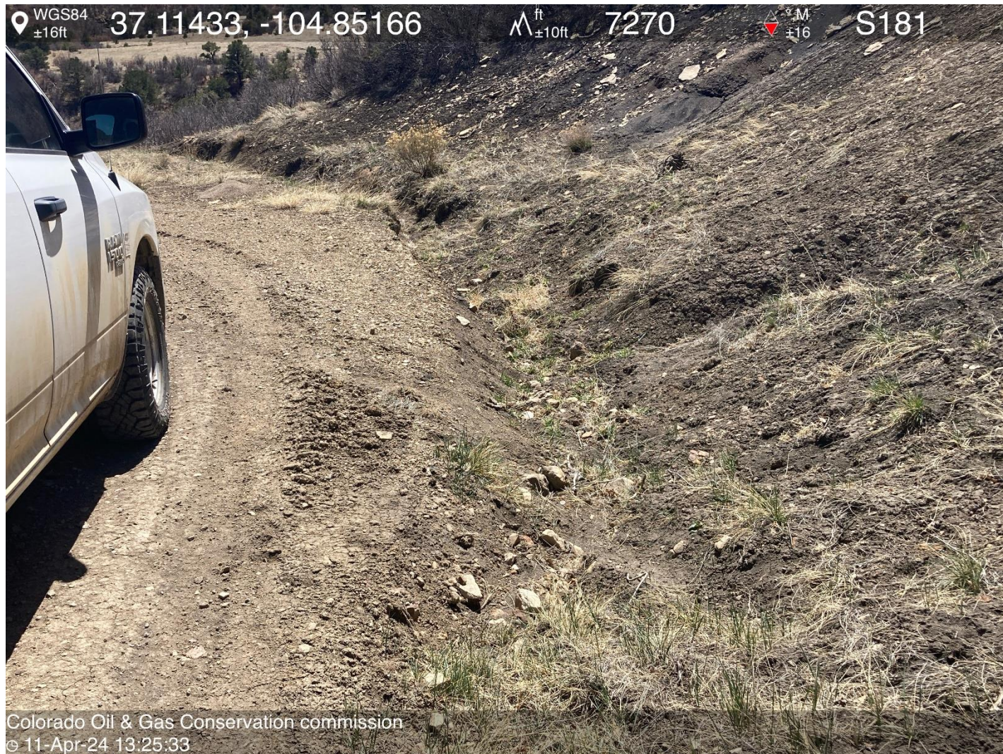
PHOTO 5: ANOTHER IMAGE OF BMP FAILURE NOTED IN PREVIOUS PHOTO.
