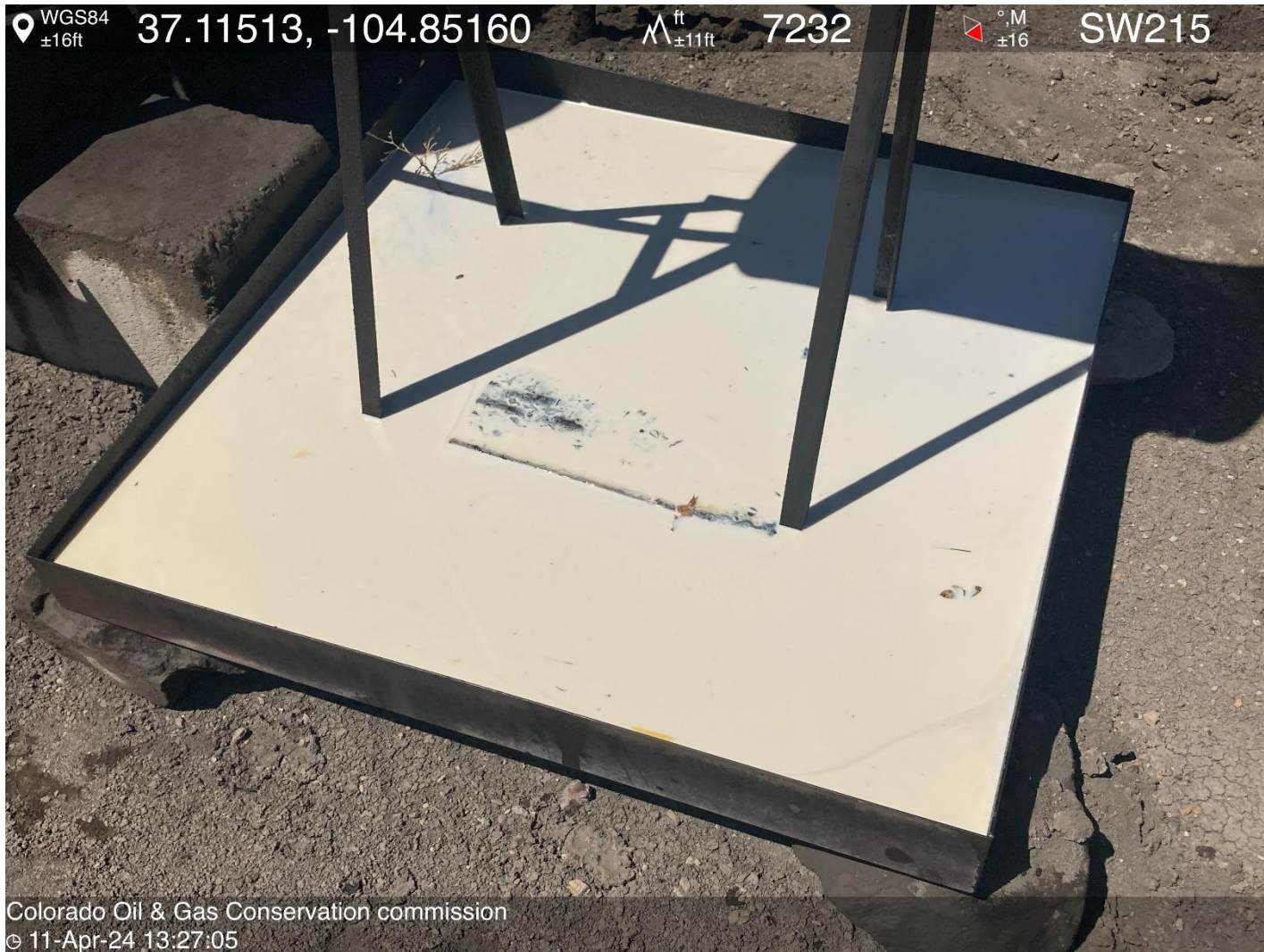
PHOTO 6: OILY WASTE IN OILER SECONDARY CONTAINMENT IS CLOSE TO RUNNING OVER. COMPLY WITH RULE 1002.f.(2)B, Comply with general provisions of the oil and gas act for wildlife protection AND SB-181. IMMEDIATE ACTION IS REQUIRED. CA DATE 4-12-2024.
