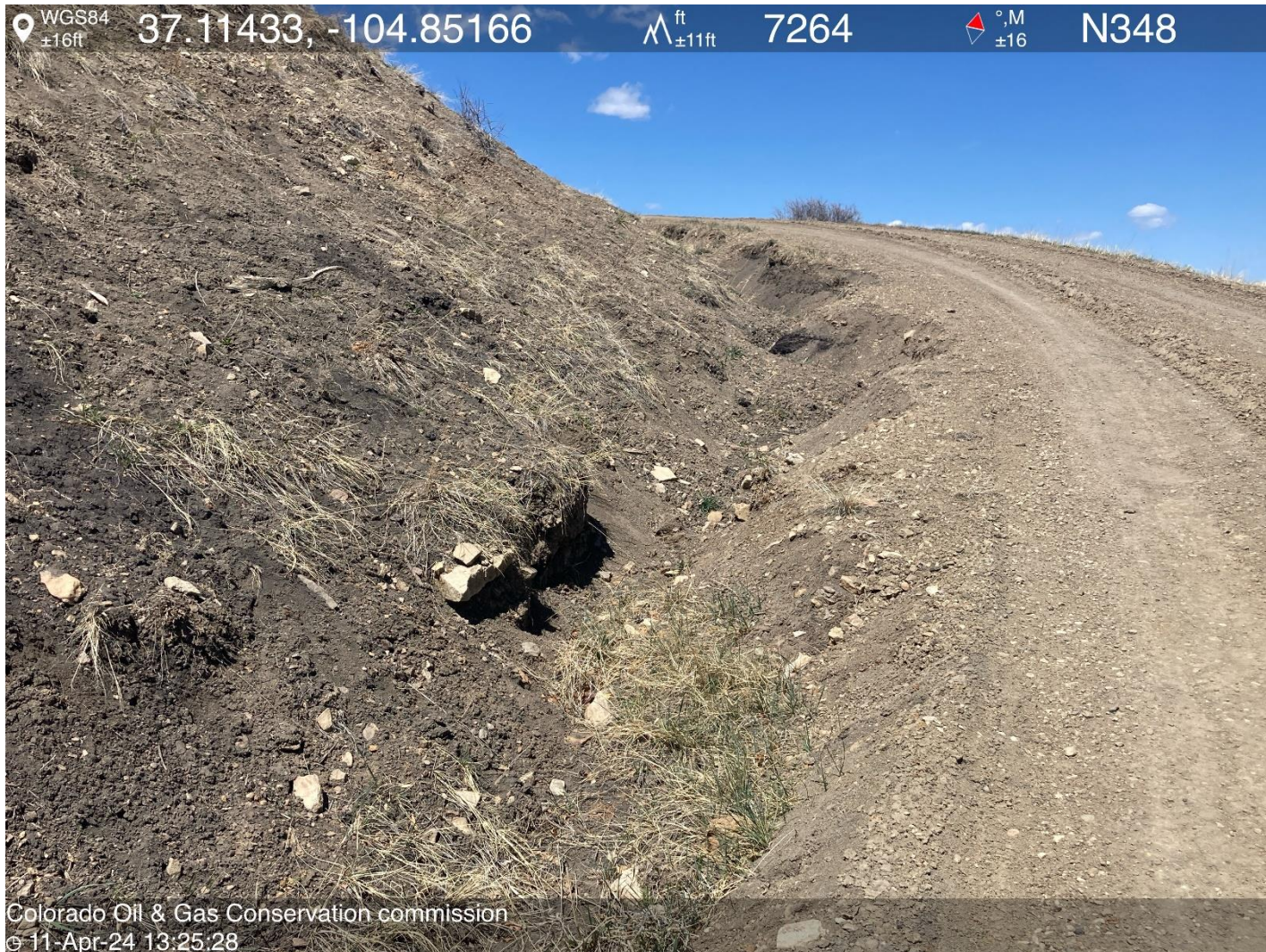
PHOTO 4: LACK OF BMP'S OR BMP FAILURE HAS RESULTED IN SEDIMENT WASHING DOWN THE ROW BMP DITCH. INSTALL OR REPAIR BMP'S AND INSPECT AT REGULAR INTERVALS TO PREVENT SEDIMENT MIGRATION PER RULE 1002. CA DATE 5-11-2024.
