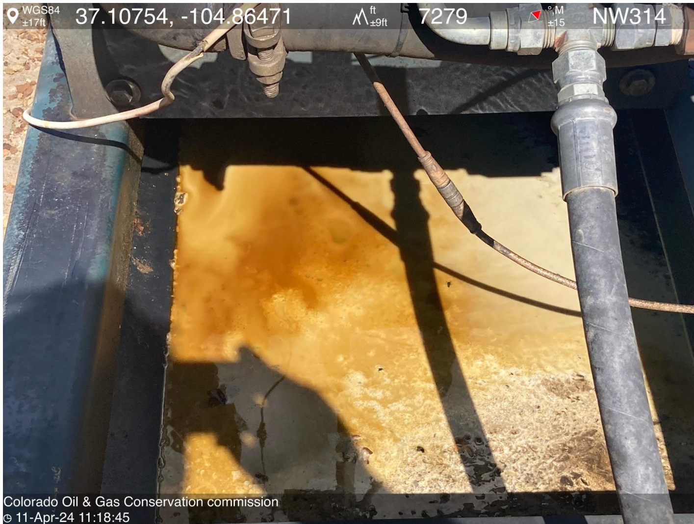
PHOTO 6: OILY WASTE IN ENGINE SKID. COMPLY WITH RULE 1002.f.(2)B, Comply with general provisions of the oil and gas act for wildlife protection AND SB-181. CA DATE 4-12-2024.
