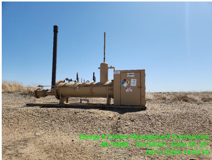
Photo 7 Horizontal Heated Separator.
