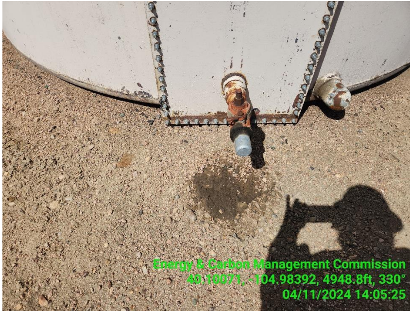
Photo 15 Stained soil by a capped leaking valve on the crude tank.
