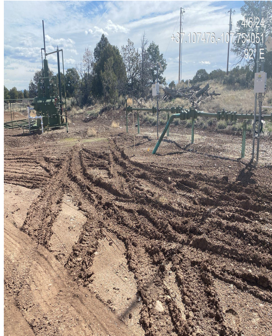
Photo 2. View of rutting/storm water issues observed on location. Additional stabilization is needed to minimize site degradation.
