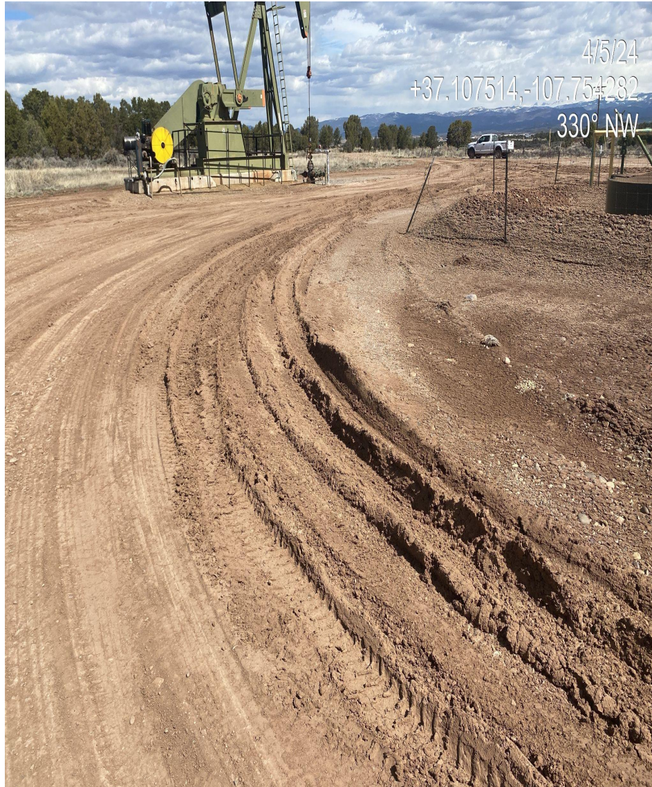
Photo 2. View of rutting/storm water issues observed on location. Additional stabilization is needed to minimize site degradation.
