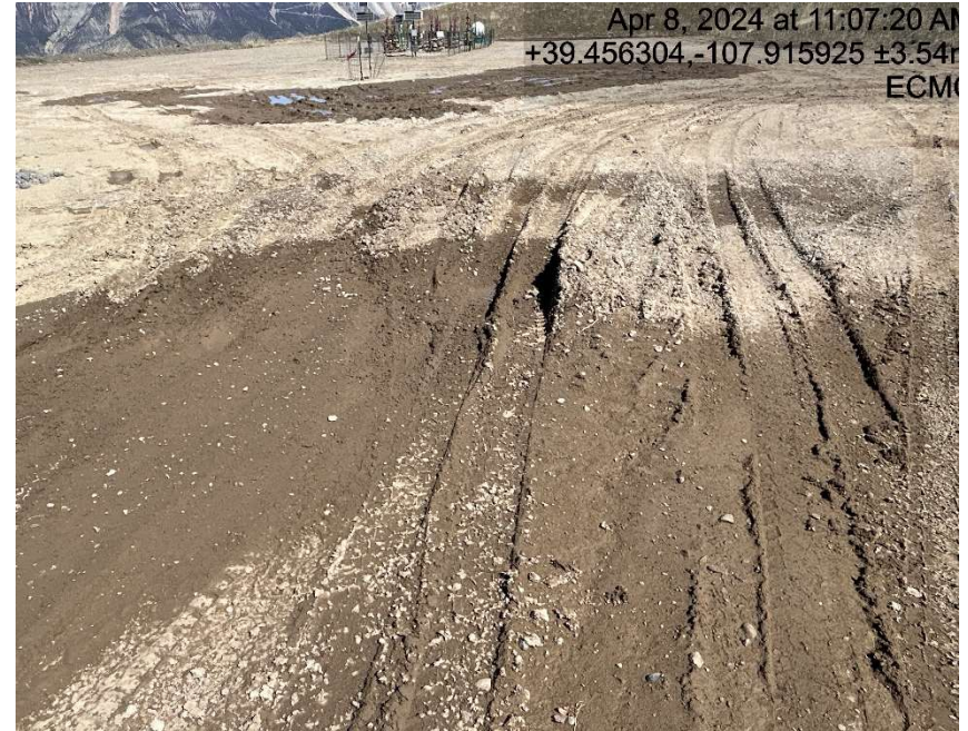
Lack of stabilization/compaction
