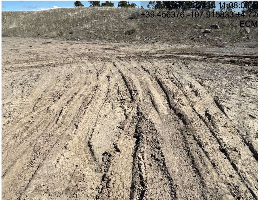
Lack of stabilization/compaction
