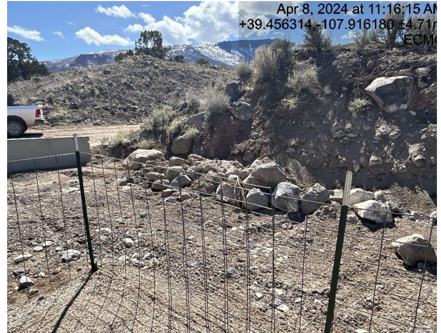
Lack of stabilization/compaction/erosion
