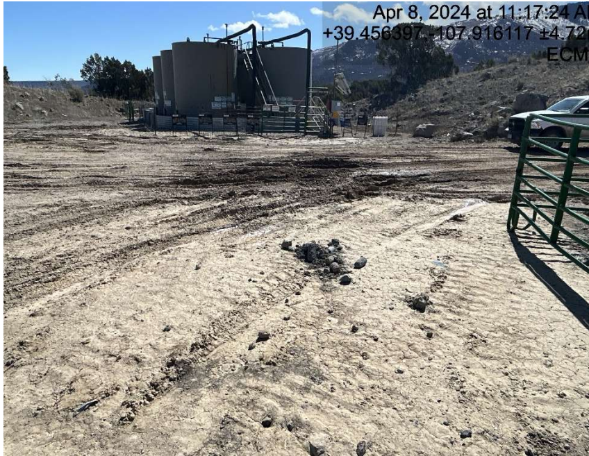
Lack of stabilization/compaction
