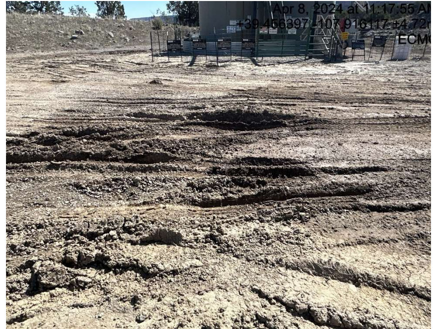
Lack of stabilization/compaction
