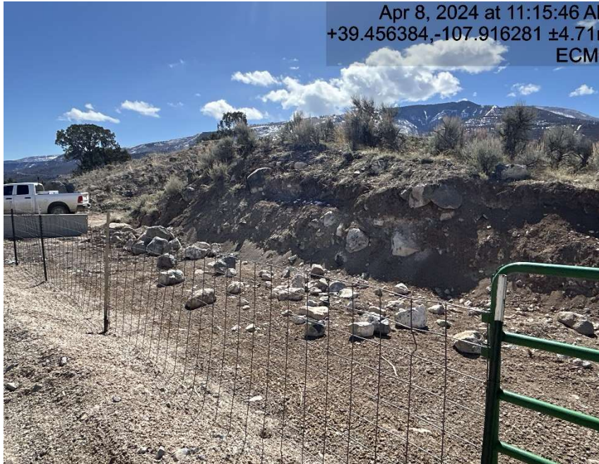
Lack of stabilization/compaction/erosion
