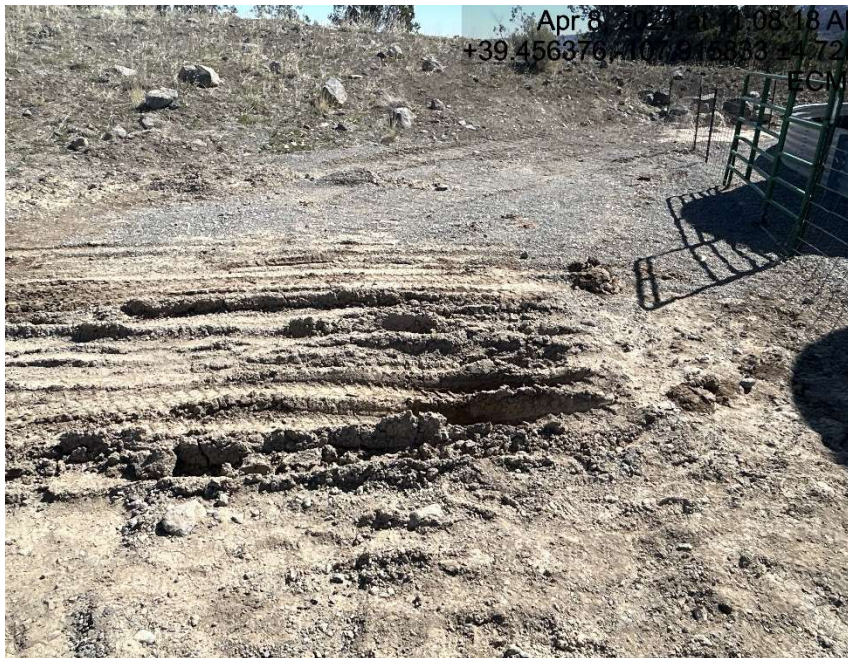
Lack of stabilization/compaction
