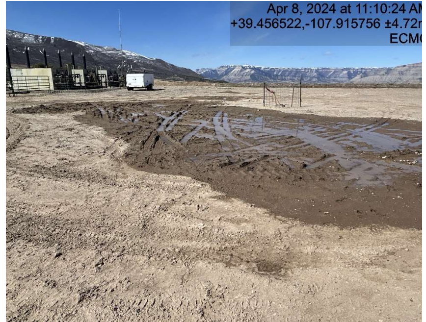
Lack of stabilization/compaction
