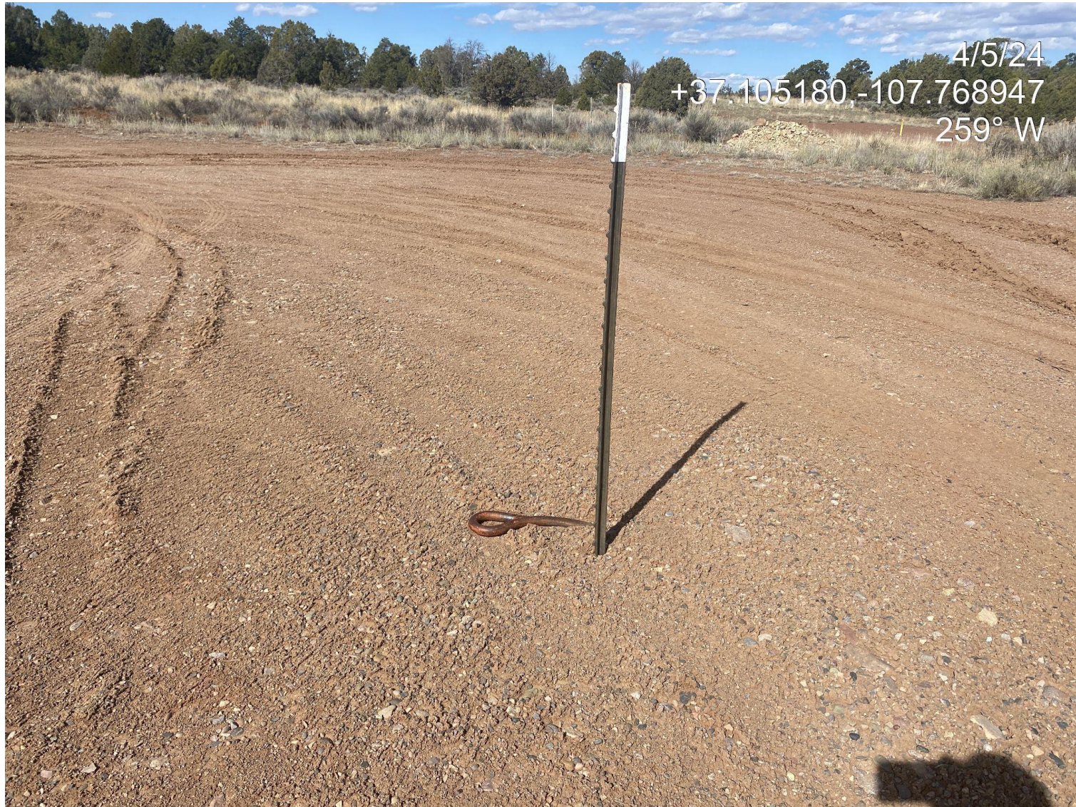
Photo 3. Unmarked guy line anchor corrective action identified in the previous inspection doc #712700710 has been addressed/resolved.
