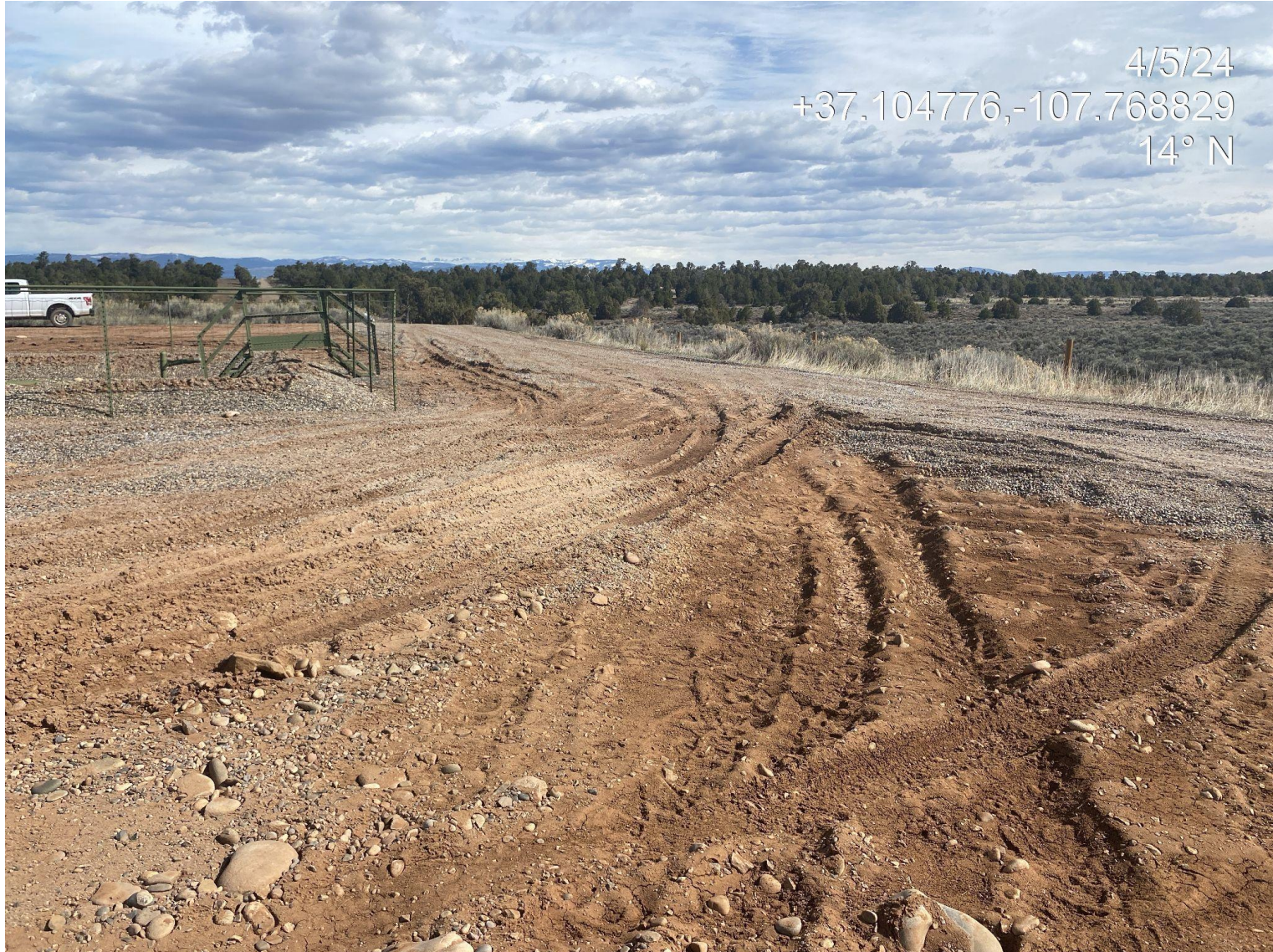
Photo 4. Rutting observed location wide. Additional stabilization is needed to minimize site degradation.
