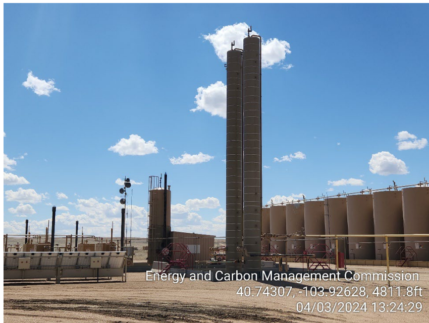
Photo 7 – VRTs and Heater Treater
