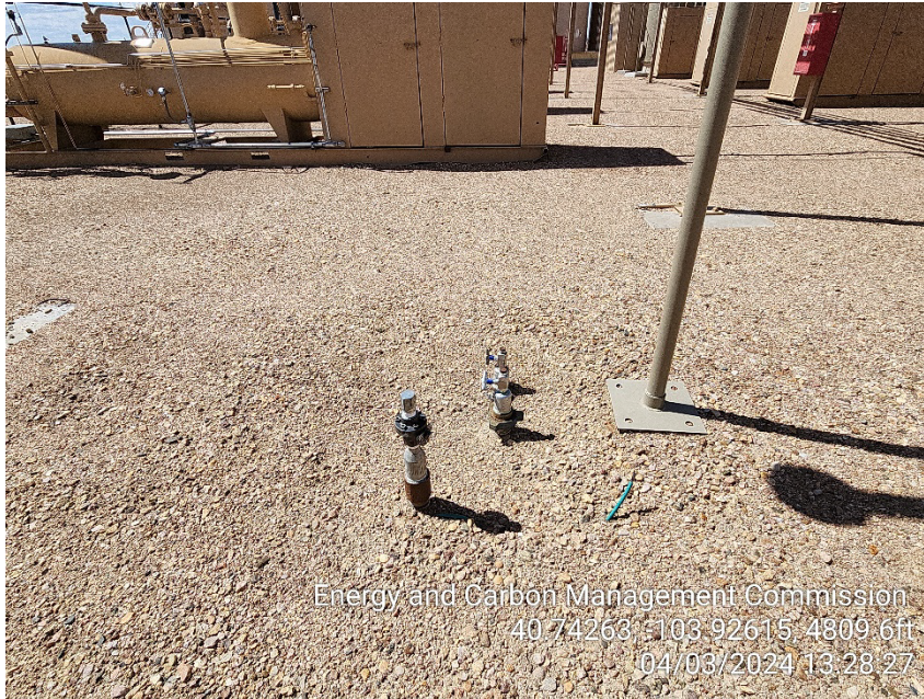
Photo 15 – Unmarked Risers at Separators
