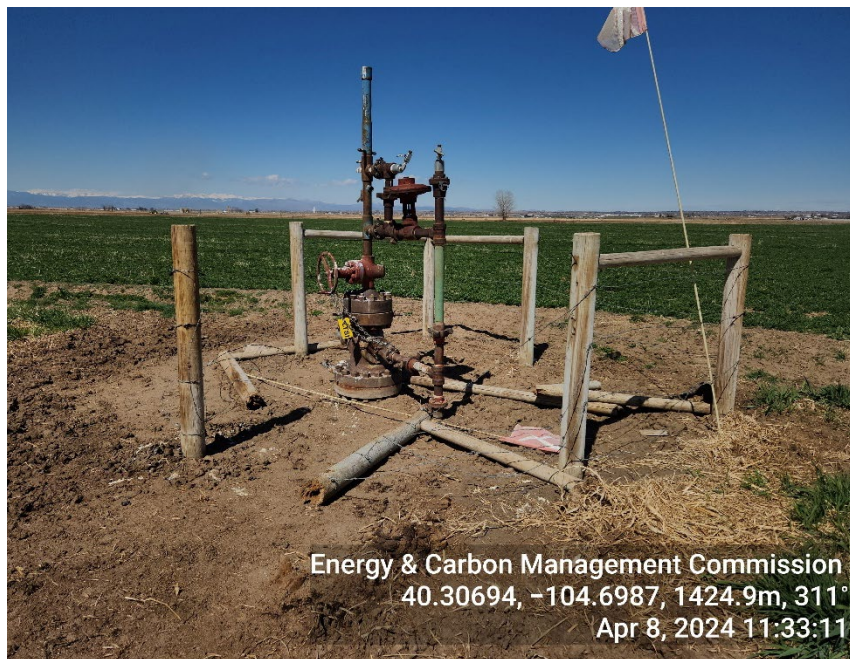
Photo 1: Wellhead, no signage, damaged fencing.
