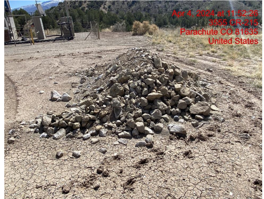
Unprotected Soil Stockpile – Photo #00423
