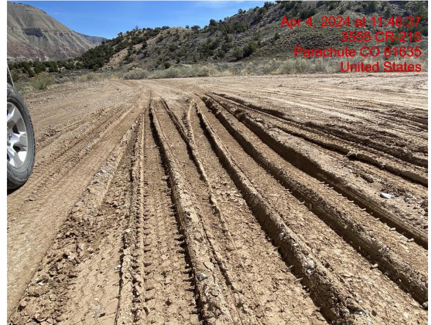
Lack of Stabilization/Insufficient Vehicle Tracking BMPs at Location Entrance/Exit – Photo #00416
