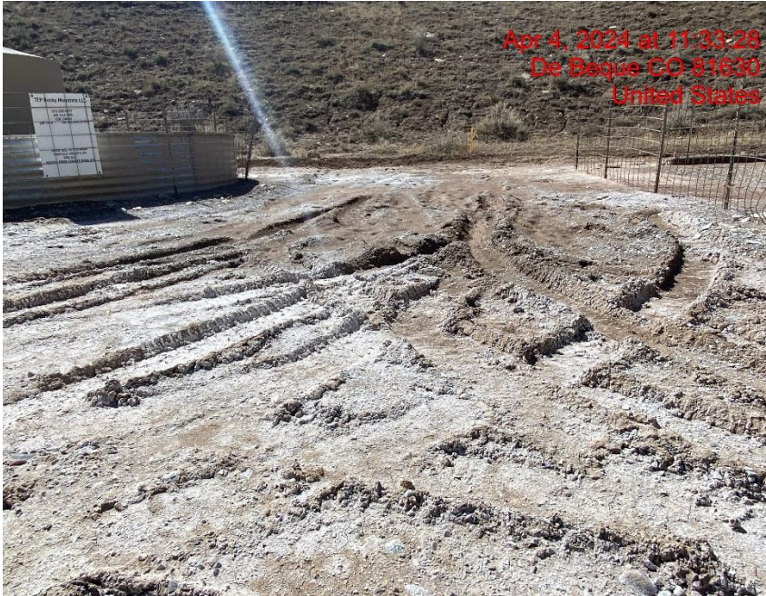
Lack of Stabilization – Photo #00403
