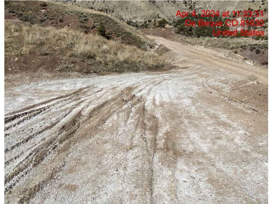
Insufficient Vehicle Tracking BMPs at Location Entrance/Exit – Photo #00404
