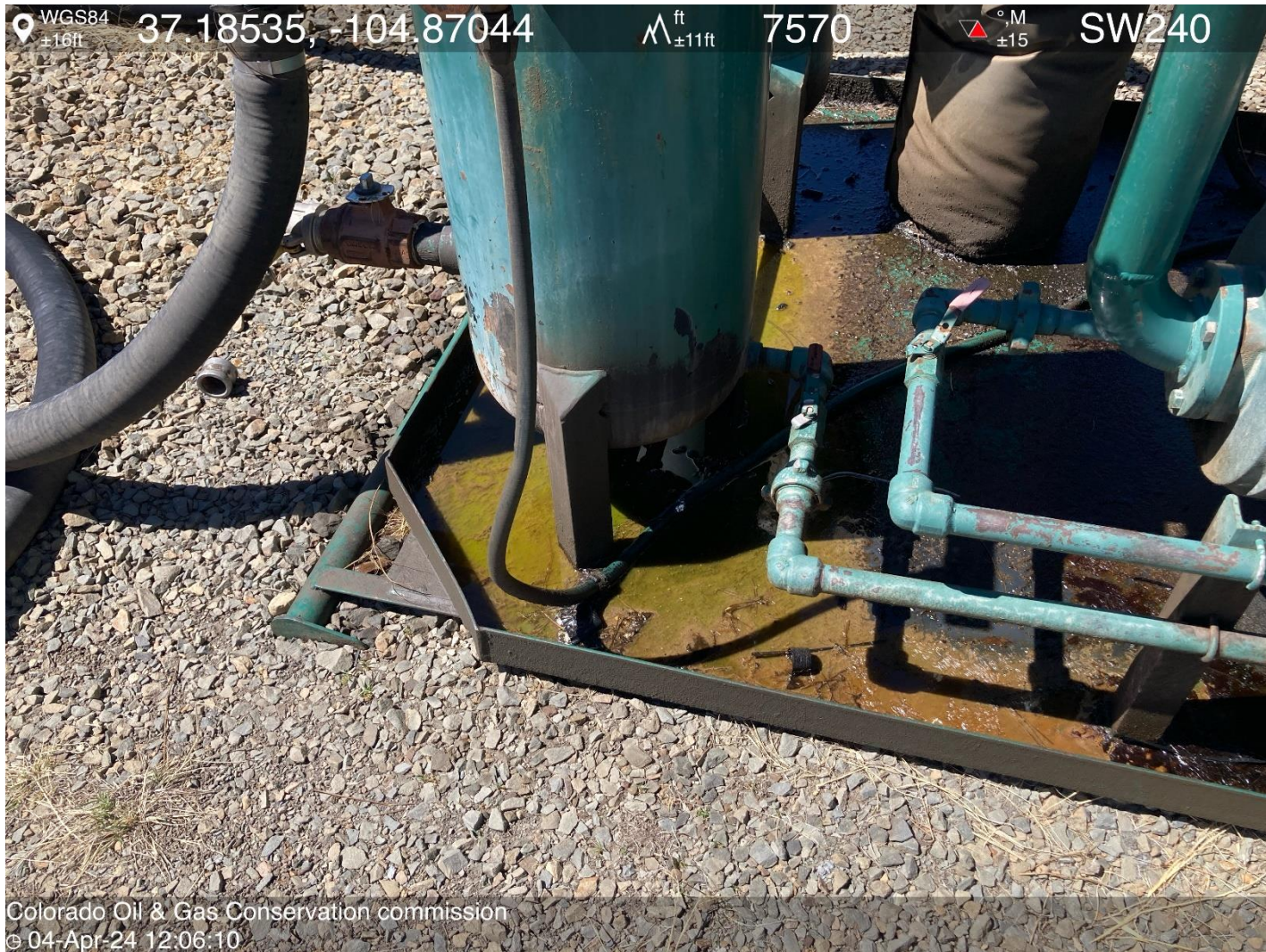
PHOTO 5: OILY/ANTI FREEZE WASTE IN TR WELL COMPRESSOR SKID. COMPLY WITH RULE 1002.f.(2)B, Comply with general provisions of the oil and gas act for wildlife protection AND SB-181. CA DATE 4-5-2024.
