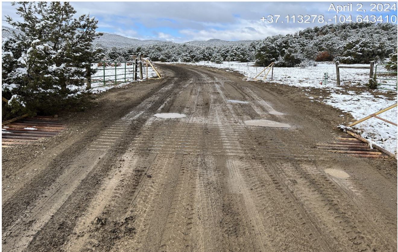
Photo 2. There are two additional cattleguards further along the road that have filled in with sediment.
