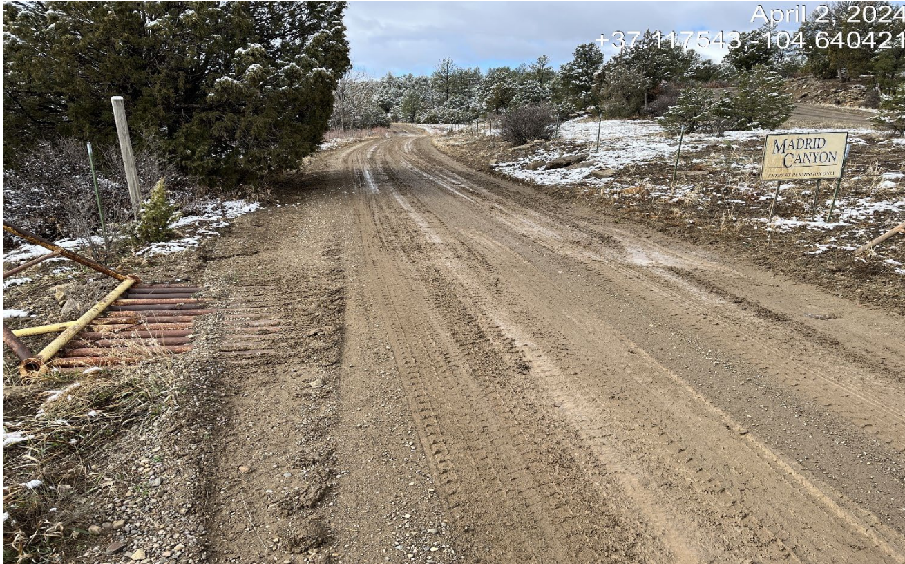
Photo 1. Facing southwest along the main access road. The cattle guard has filled in with sediment and needs to be cleaned out.
